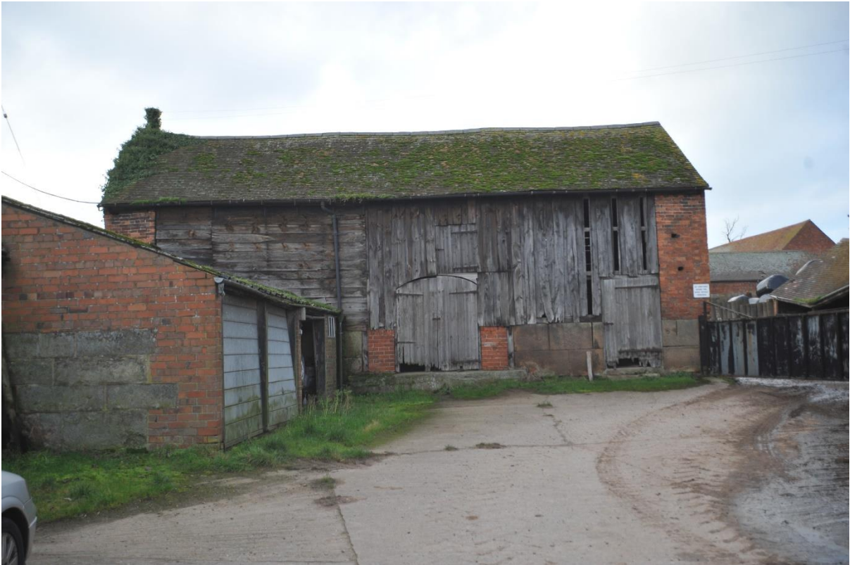
Pl.2: The east elevation of the Barn (Building A).
