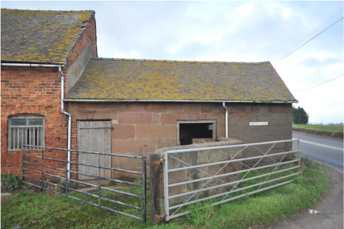
Pl.10: The south side of the Stone Range (Building C).
