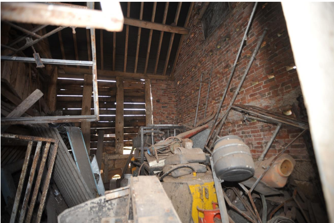
Pl.5: The little altered interior of the northern bay of the Barn.
