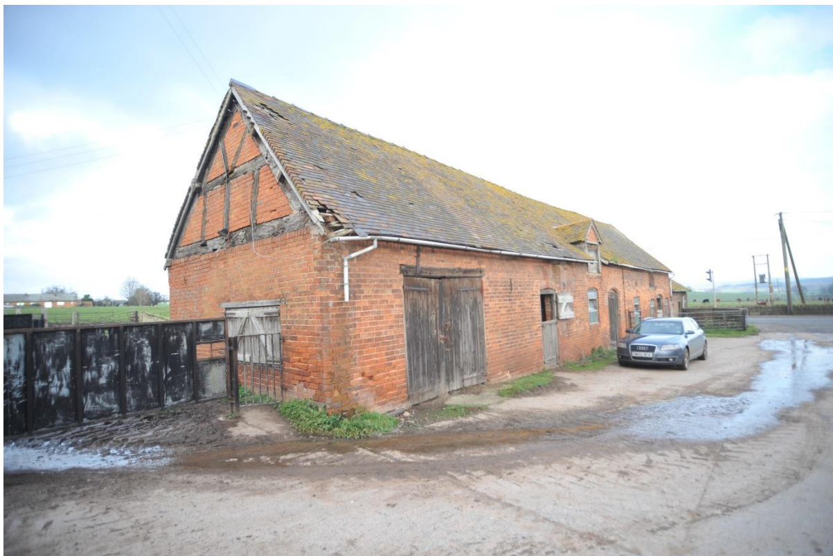
Pl.6: The Stable Range (Building B) from the south-east.
