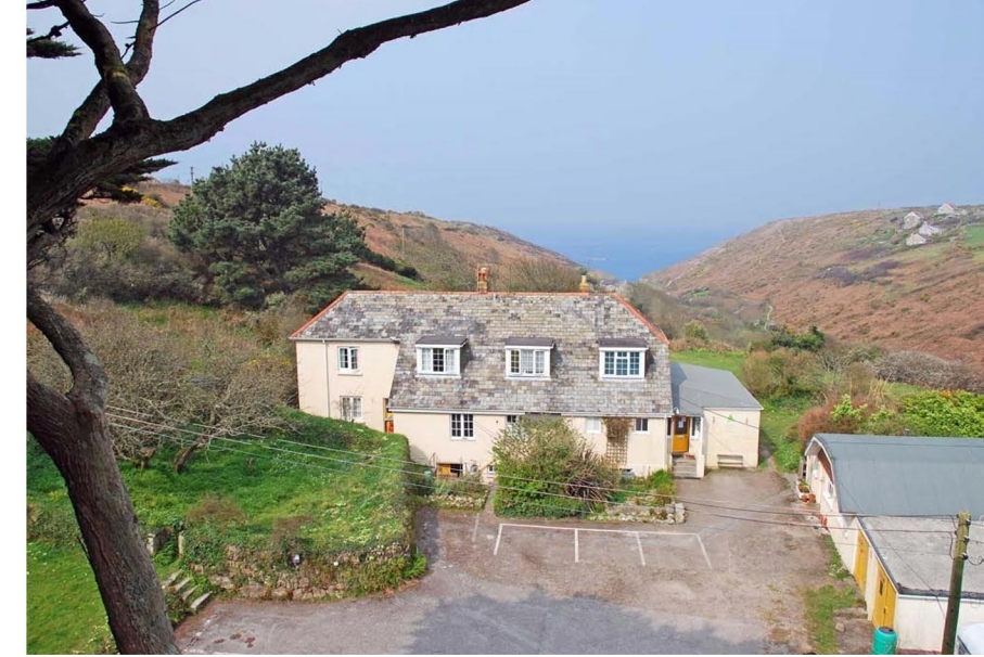
East Elevation Photo
