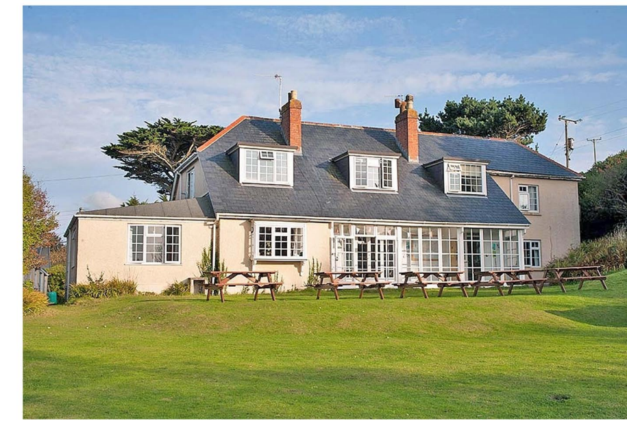
West Elevation Photo
