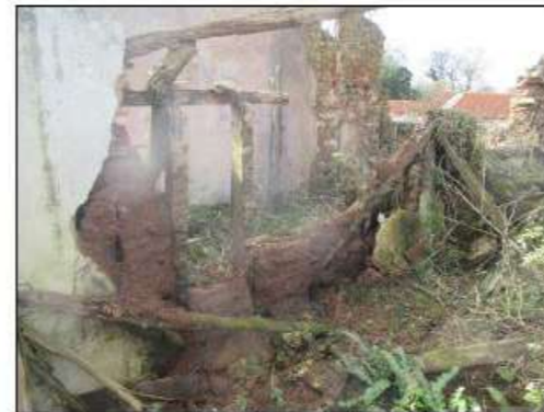
Internal timber frame wall with cob infill.
