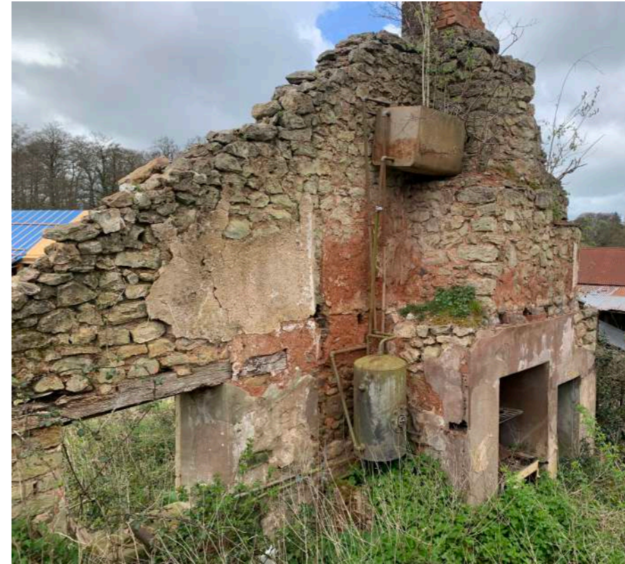
Inside face of south wall, showing details of the existing opening and chimney (04/22)
