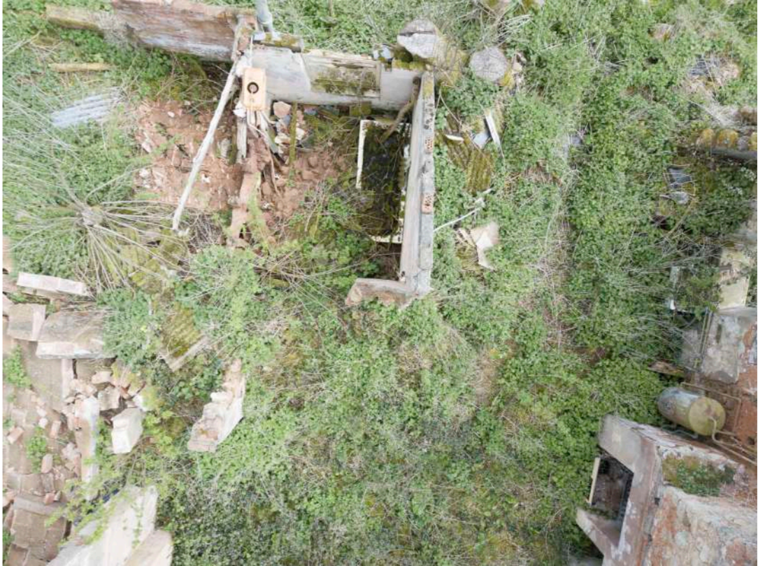
Aerial view showing remains of a former bathroom (04/22)
