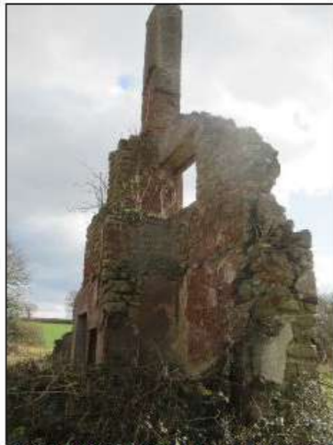
South wall, with vegetated shelves in chimney stack.
