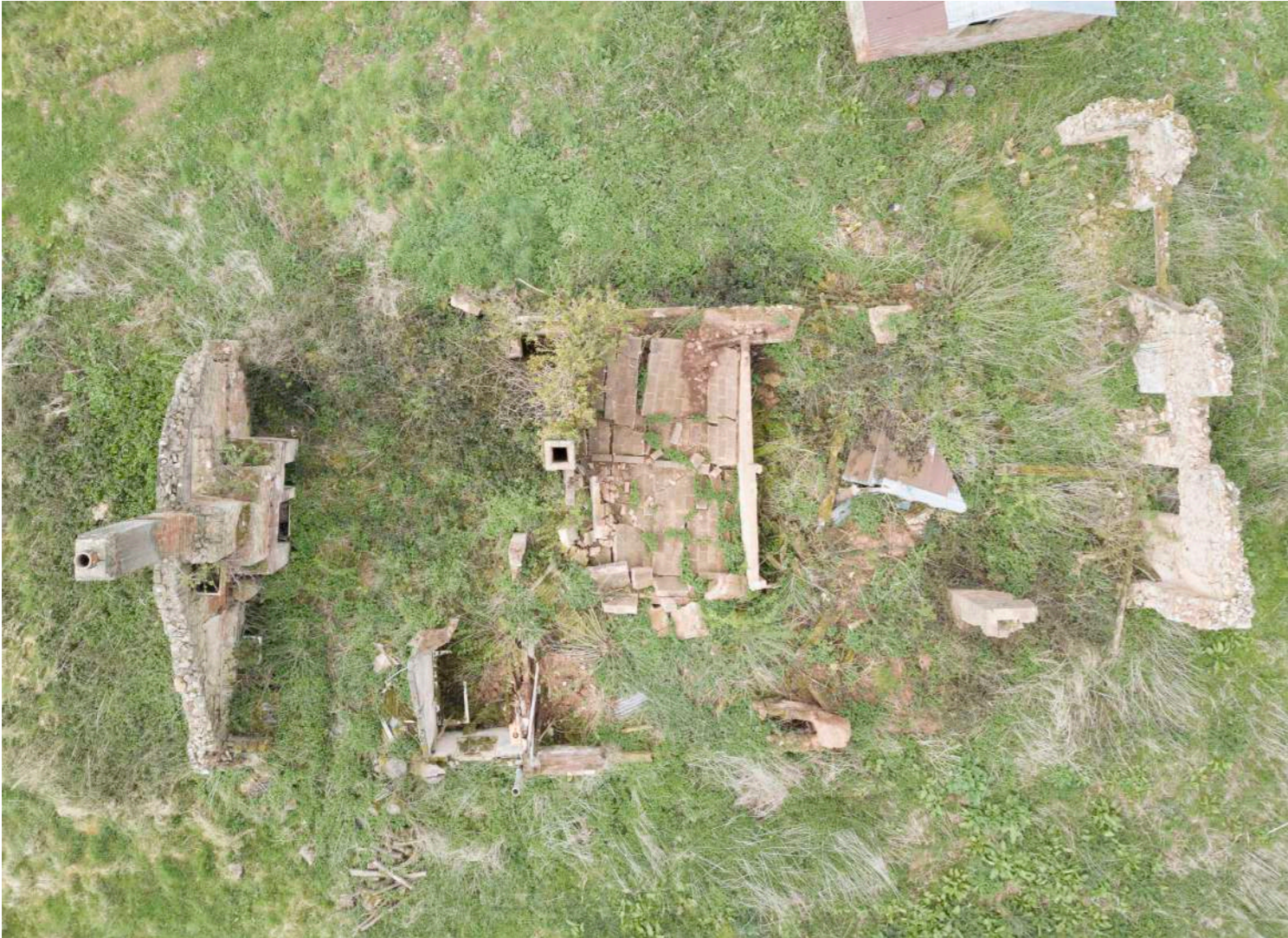
Aerial view showing remains of the structure, including collapsed walls and roof sections (04/22)
