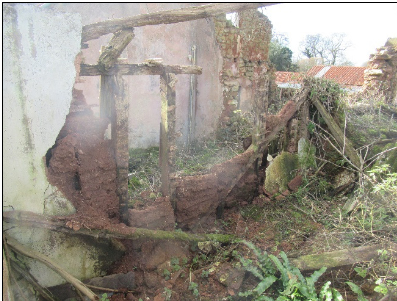
Internal timber frame wall with cob infill.
