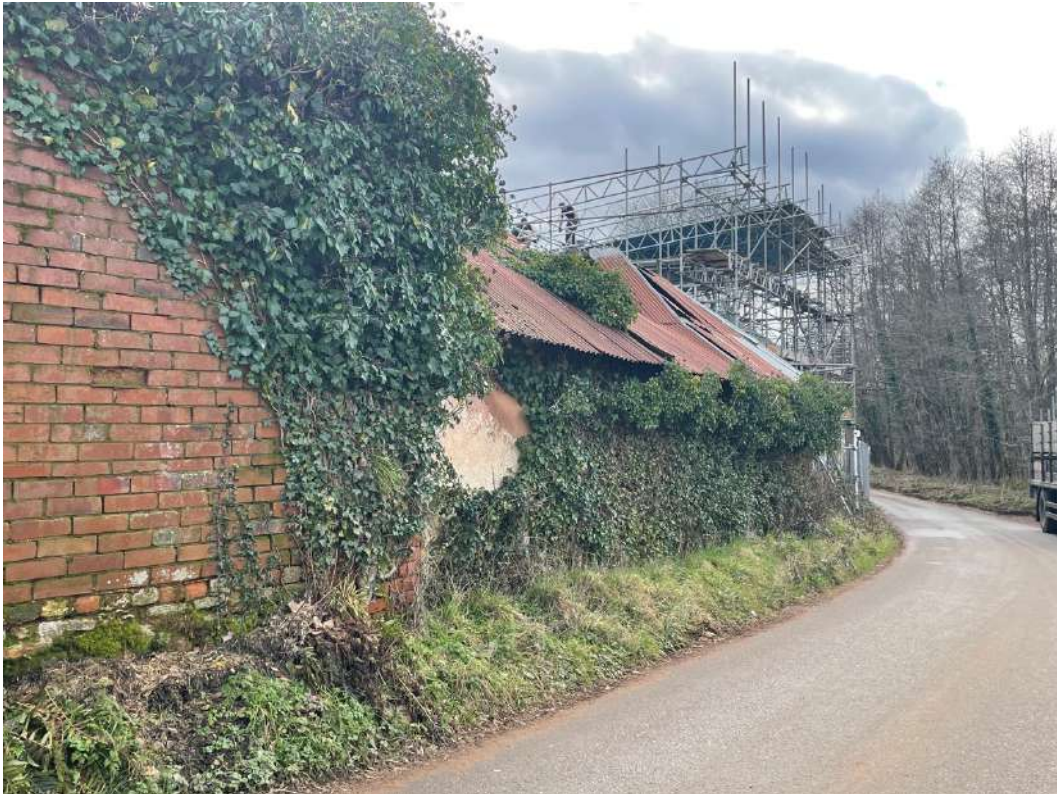
Photo 27: West elevation of Barn 2.
