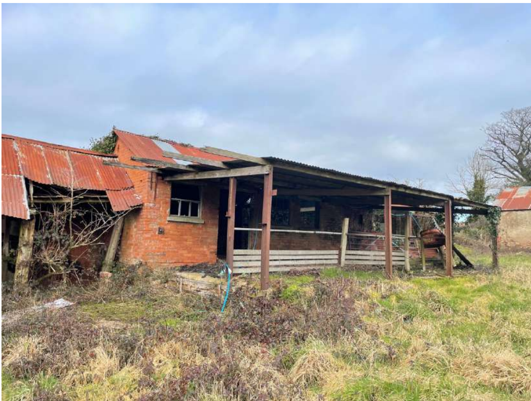
Photo 24: East elevation of Barn 2.
