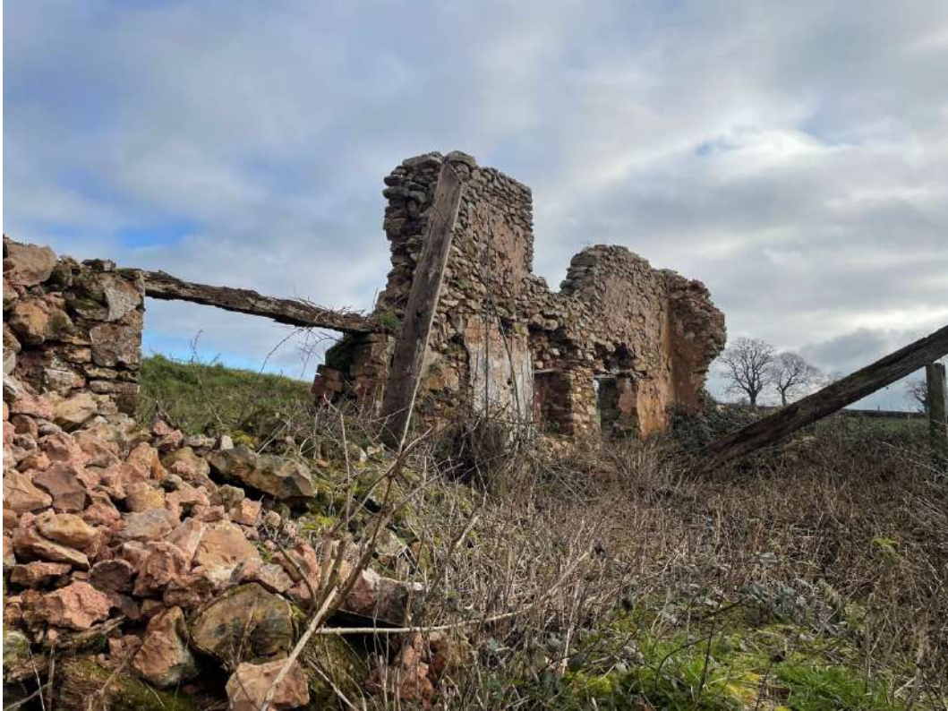
Photo 3: North wall of Farmhouse photographed from the south.
