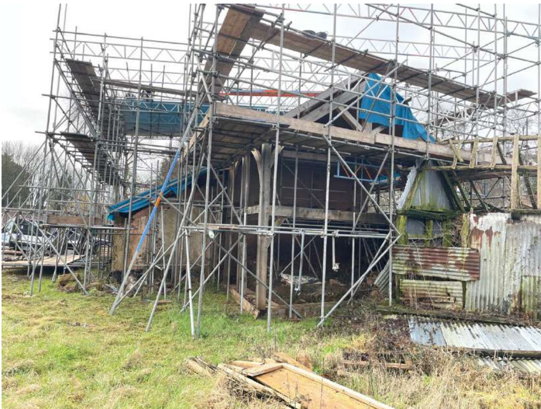
Photo 12: North elevation of Barn 1.
