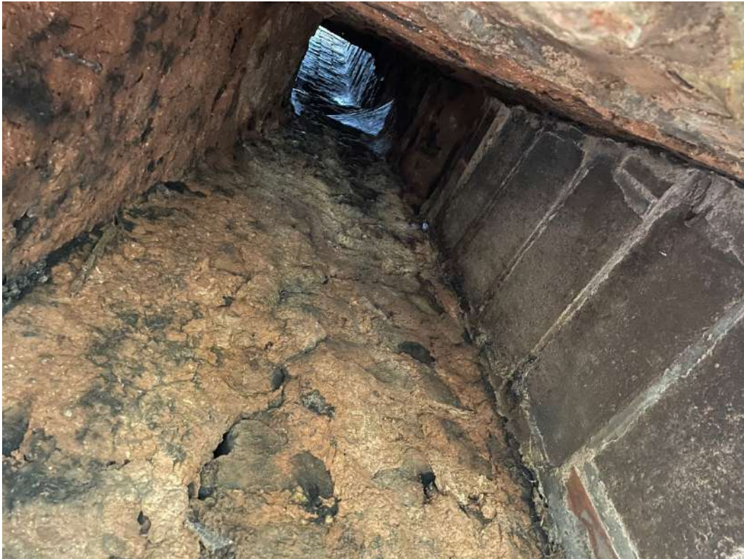
Photo 9: South chimney breast interior.
