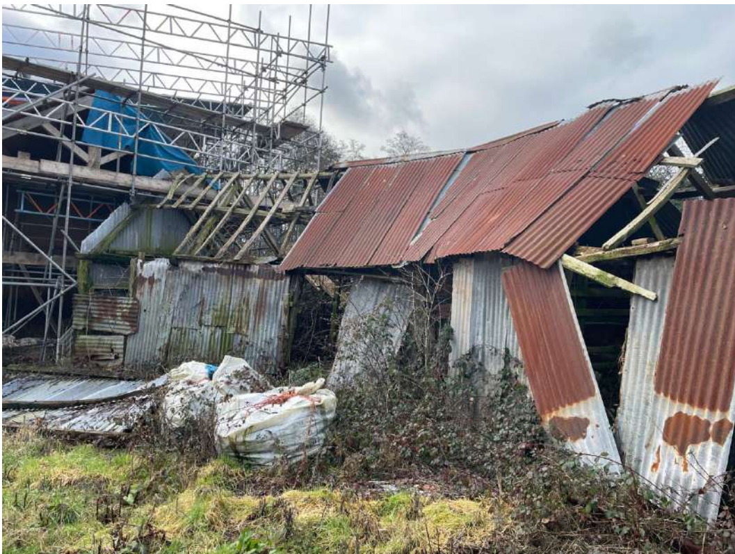
Photo 22: East elevation of Barn 2.
