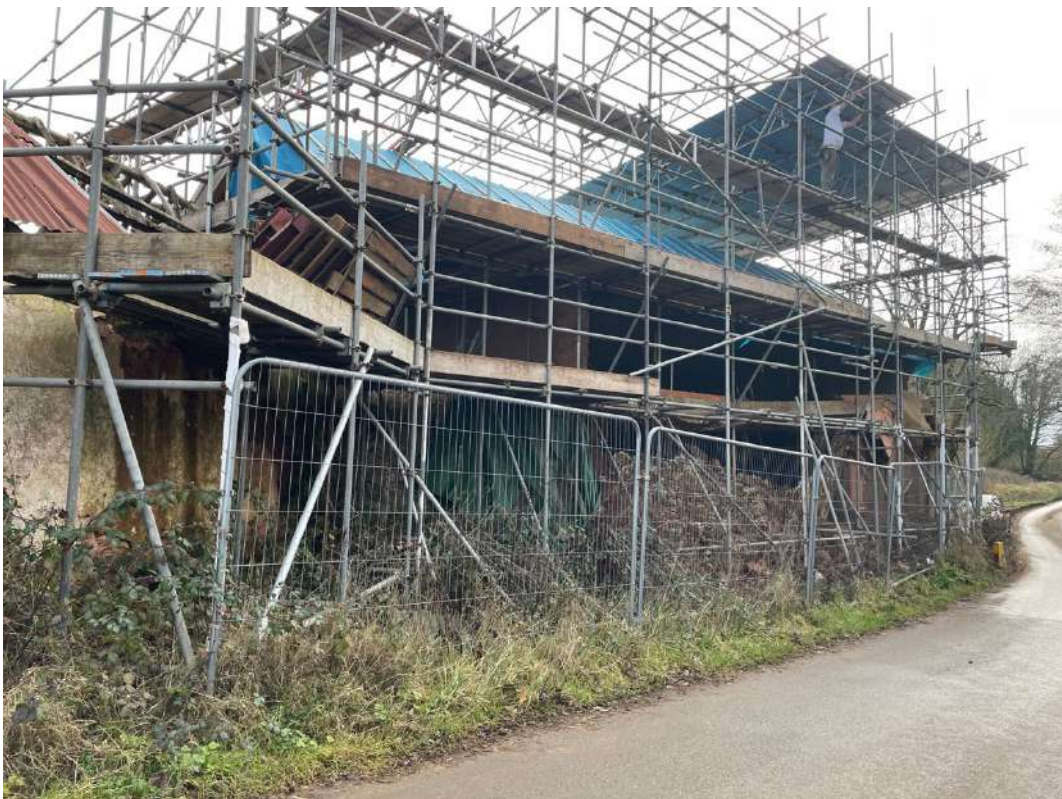
Photo 14: West elevation of Barn 1.
