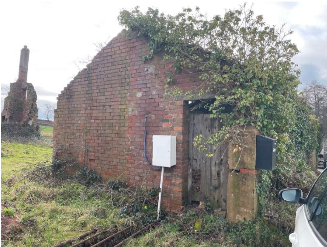
Photo 26: North elevation of Barn 2.
