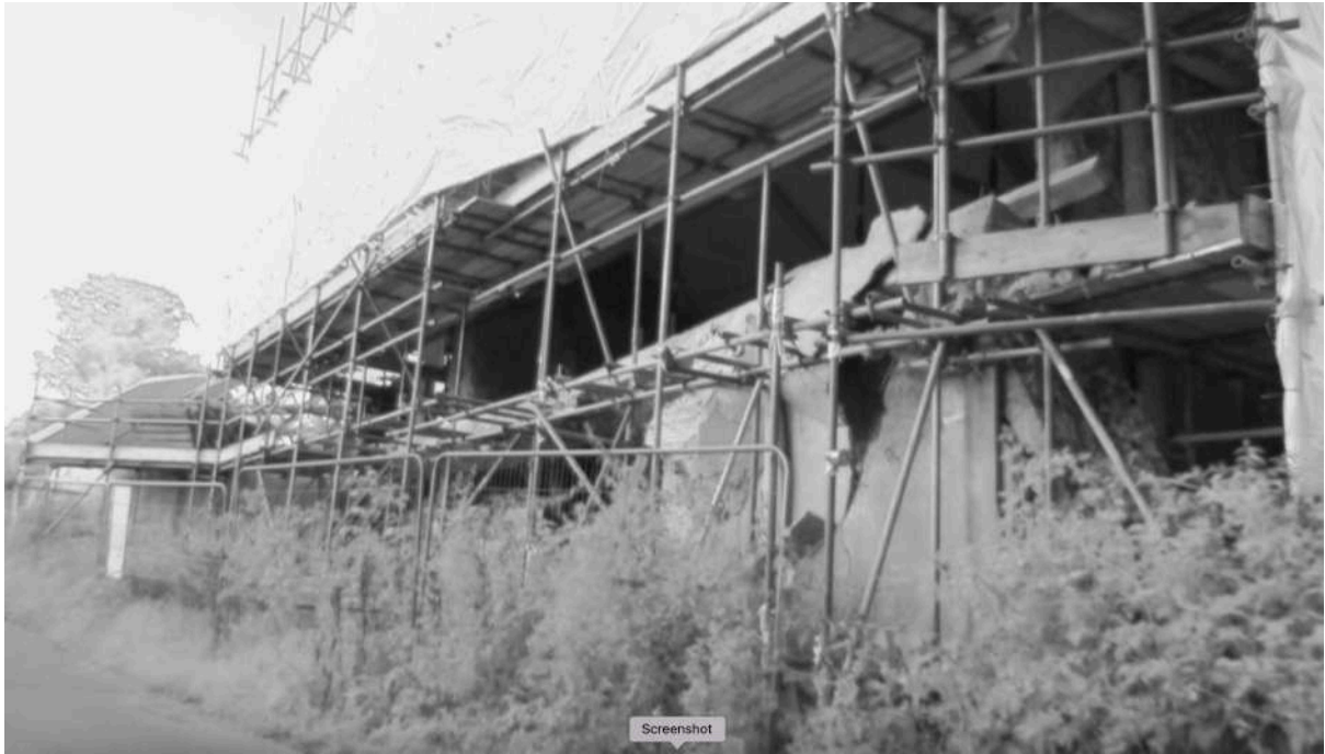
South surveyor start of survey 15.08.23
