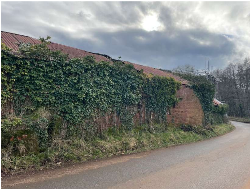
Photo 28: West elevation of Barn 2.
