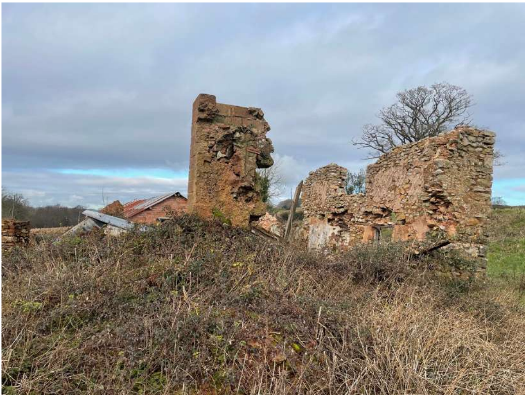
Photo 4: North wall of Farmhouse photographed from the east.
