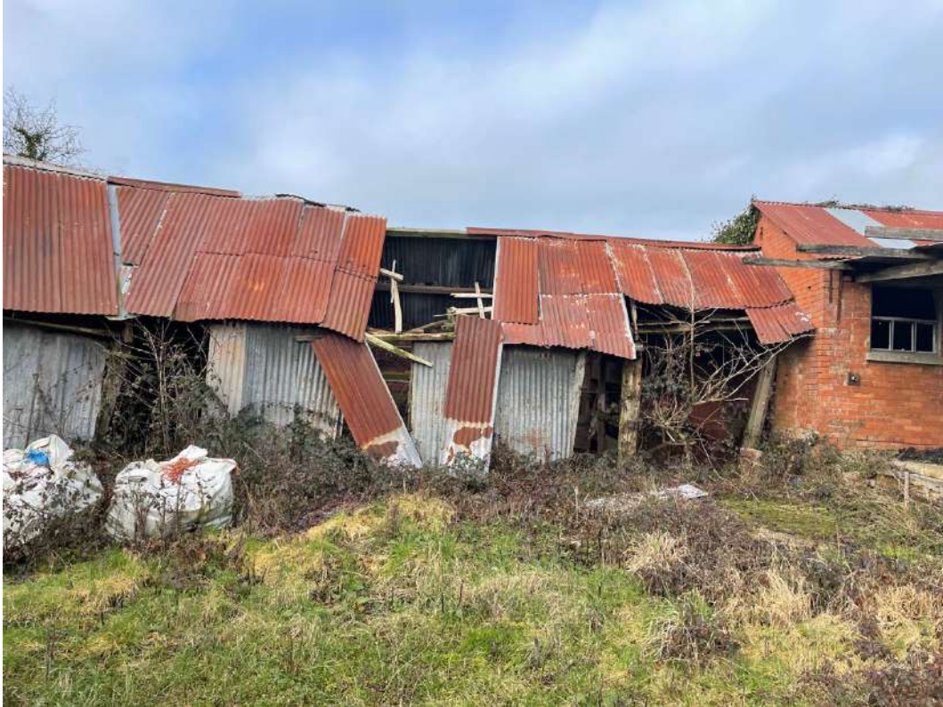
Photo 23: East elevation of Barn 2.
