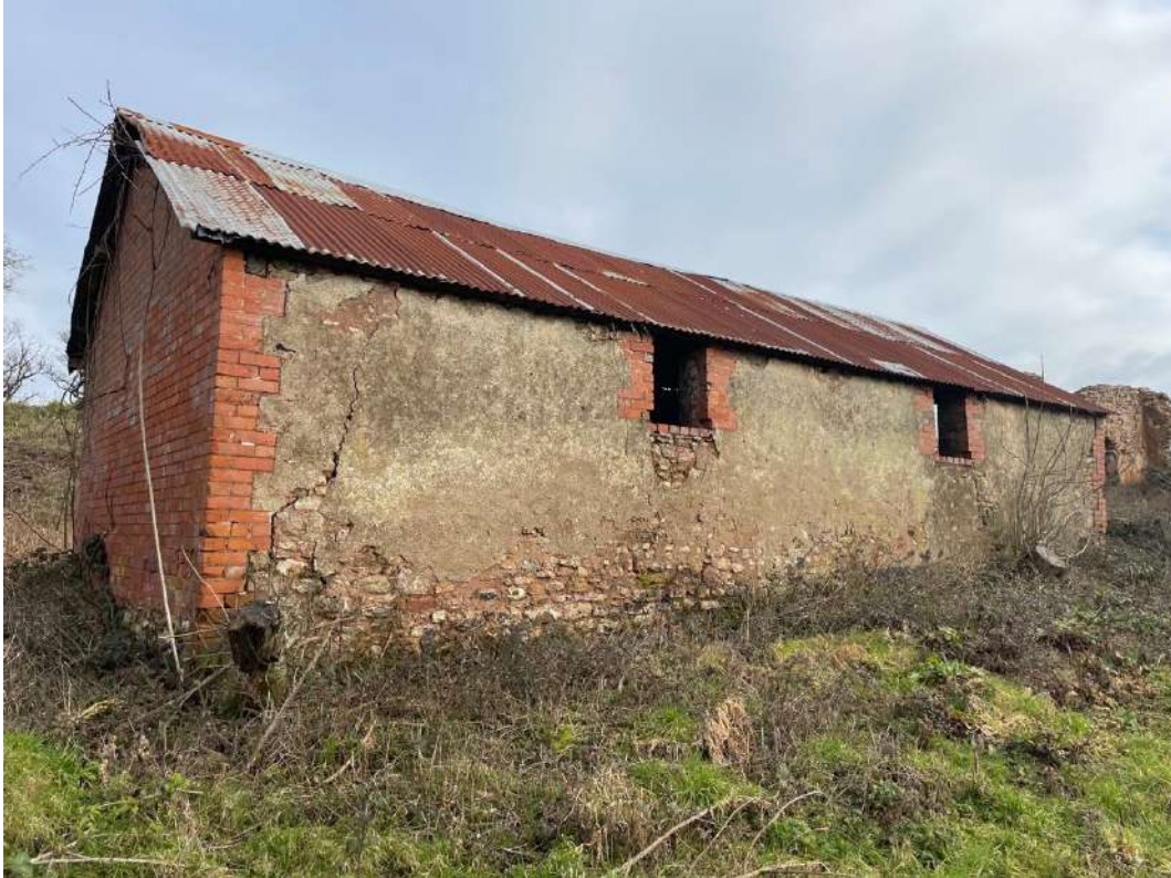
Photo 33: South and west elevations of Barn 3.
