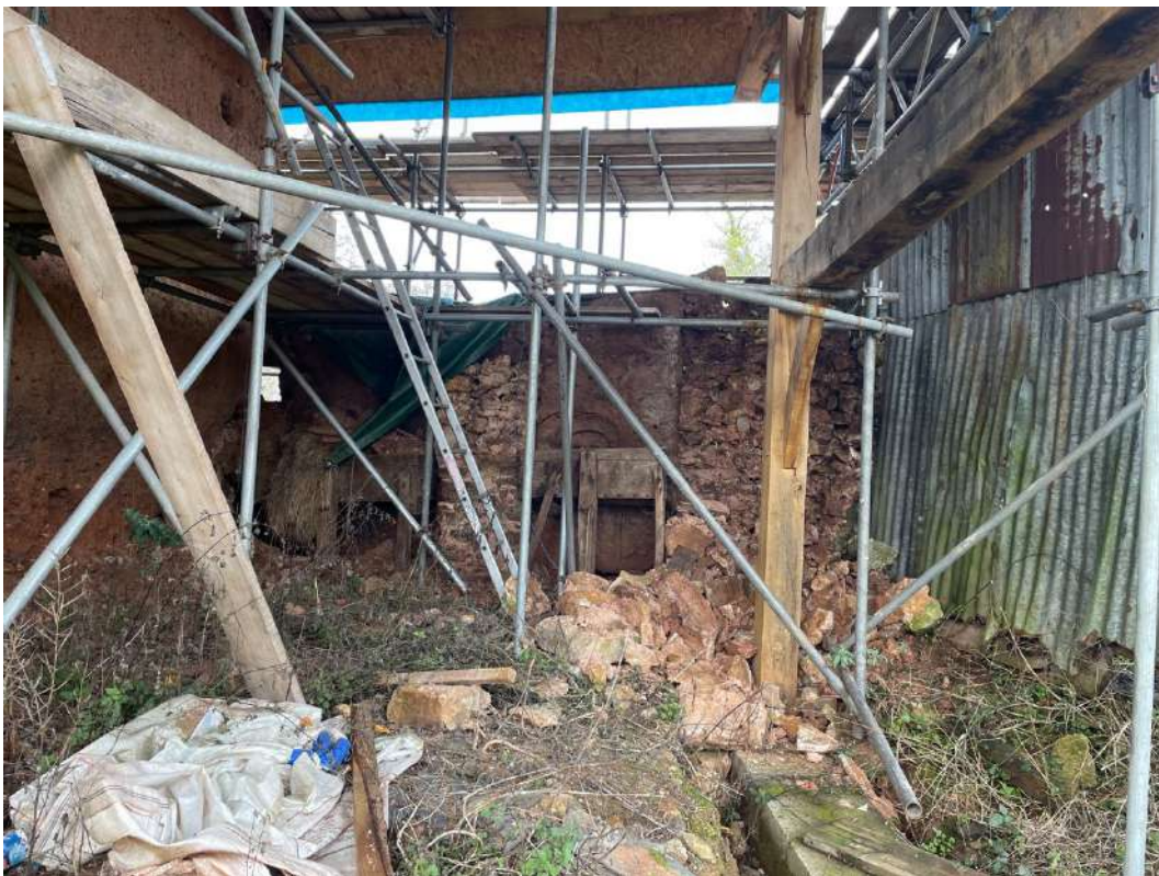
Photo 16: Barn 1 interior (to north).
