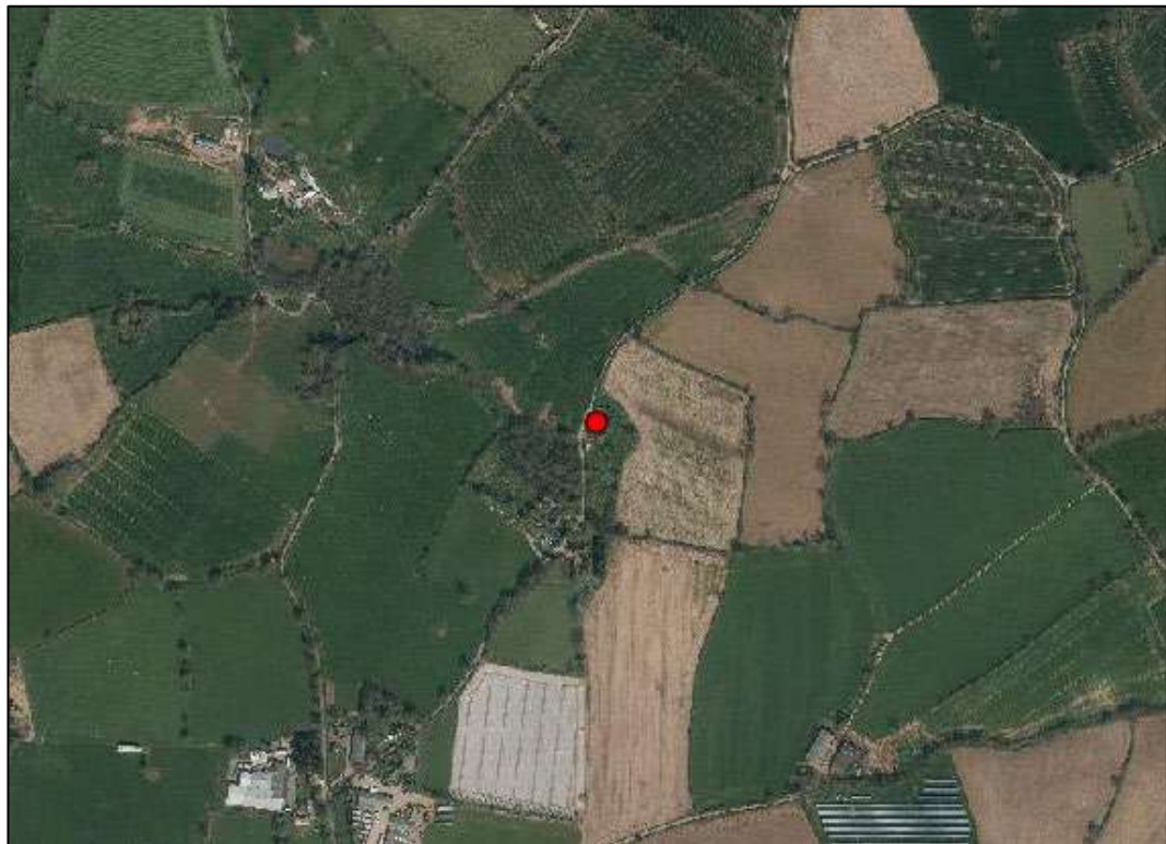
Figure 2-2: The site in the context of the surrounding landscape.
