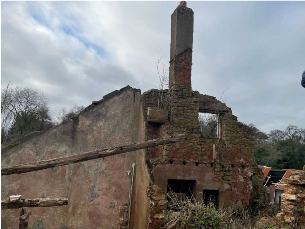
Photo 7: South wall of Farmhouse photographed from the north.
