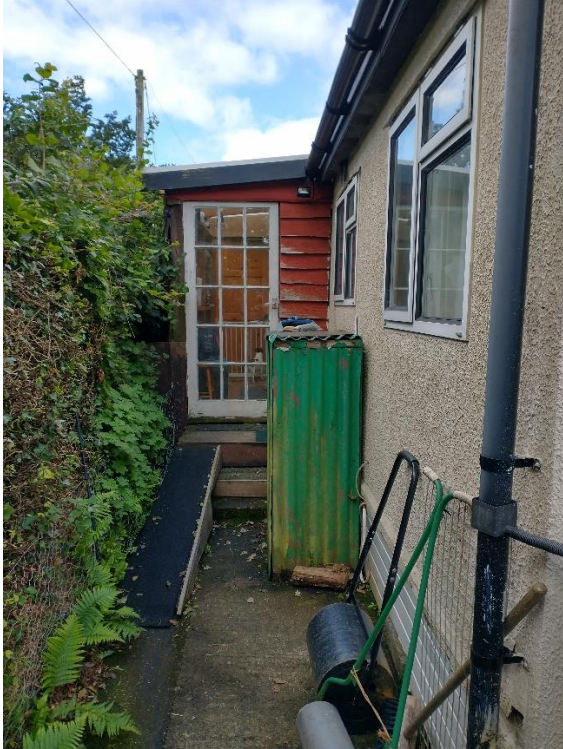
Porch as viewed from eastern end of caravan
