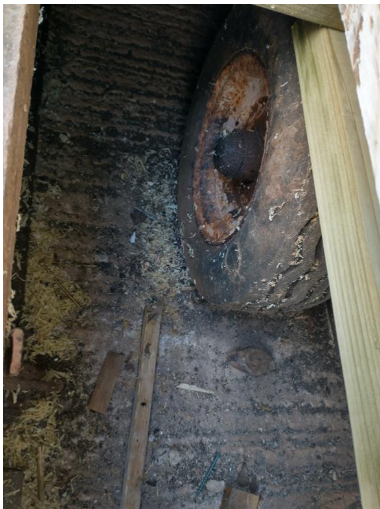
Underside of caravan on Certificate site
