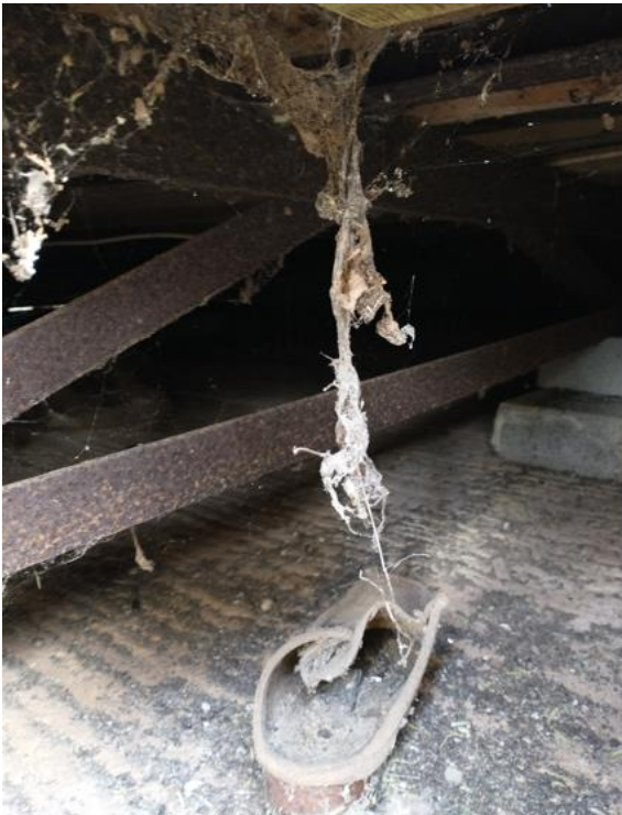
Underside of caravan on certificate site
