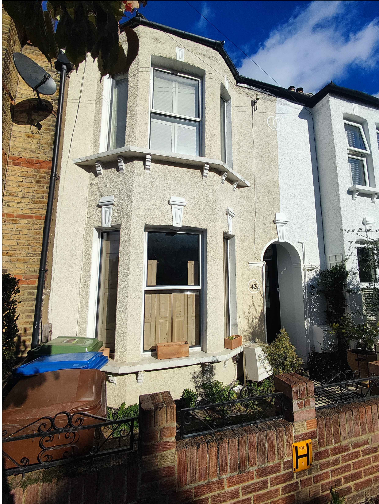
Existing front facade
