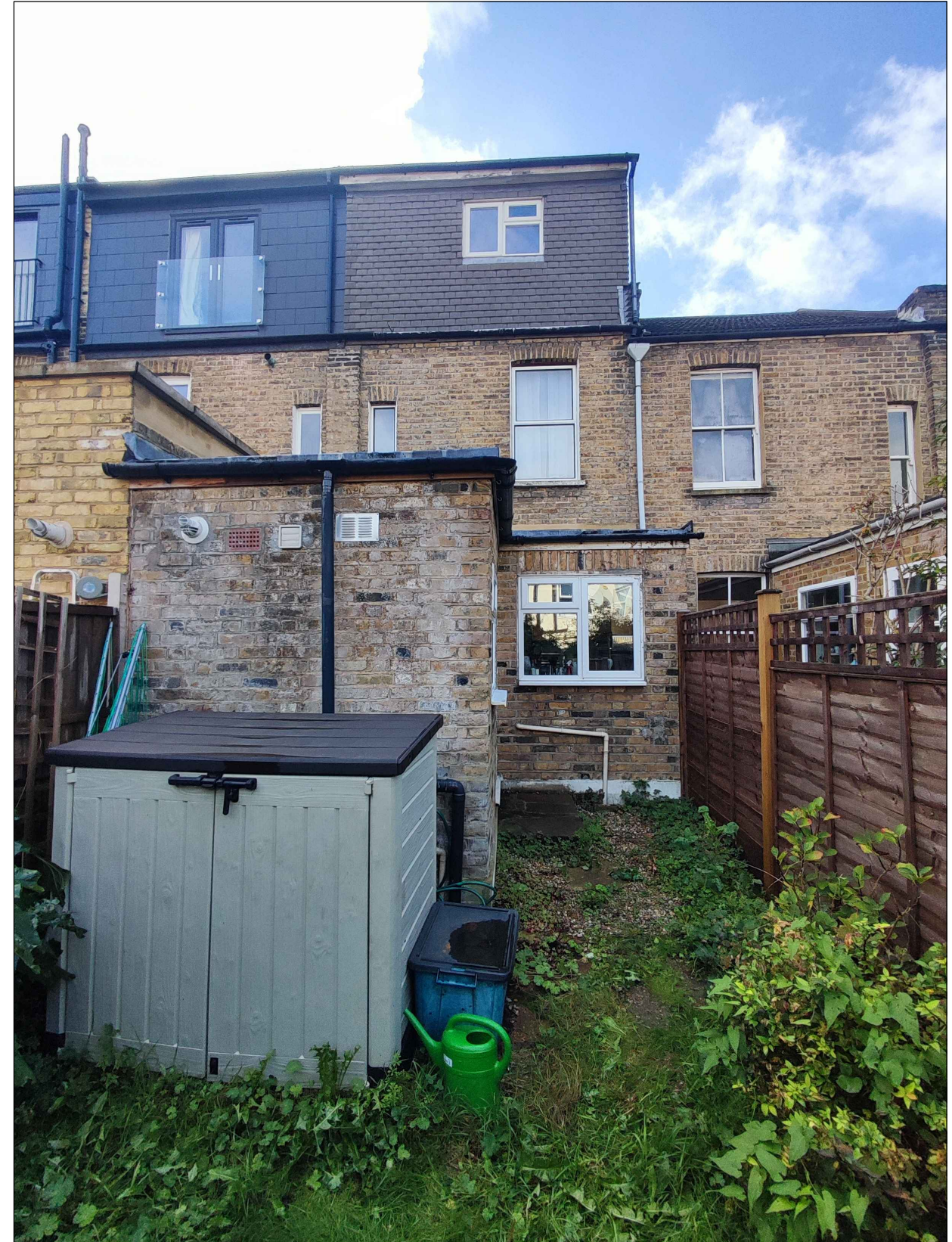
Existing rear facade
