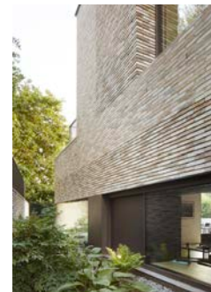
Contrasting Brick mortar joints to give elevation texture.
