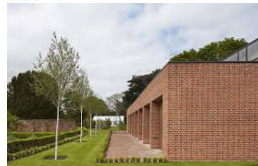
Benjamin Britten Archives by Stanton Williams Architects - simple horizontal form looks onto green space
