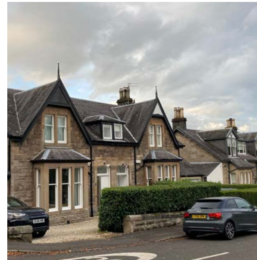
19 th century sandstone buildings defines the character of Milngavie
