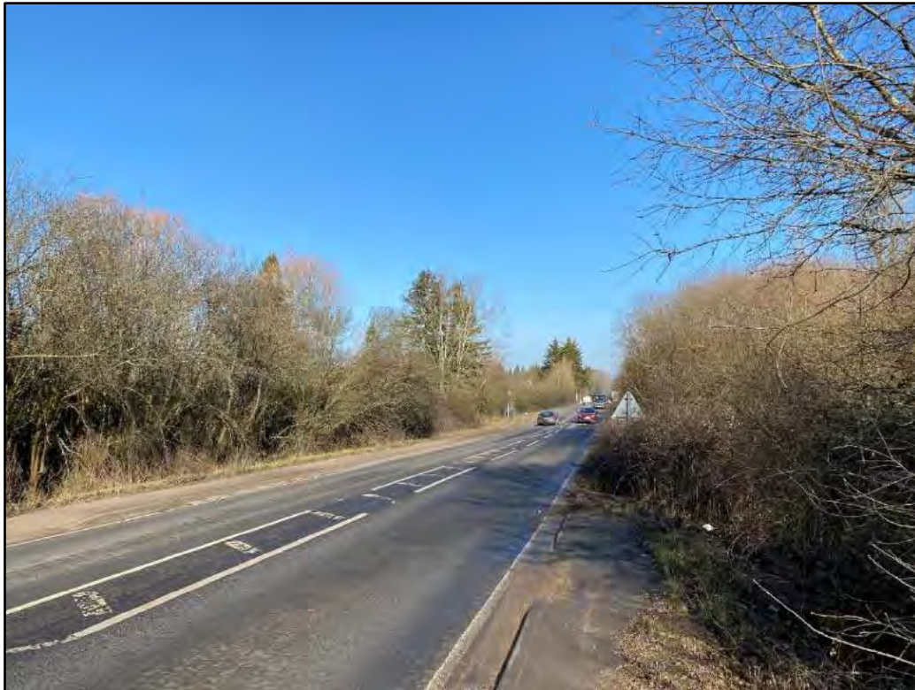
Image 2.3: Gravel Hill Road Dropped Kerb Pedestrian Crossing (Looking North)
