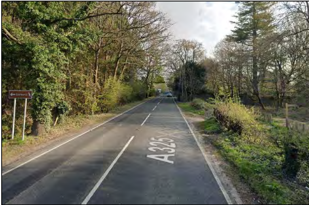
Image 2.14: Footpath 50 Connection with the A325 (Looking North)
