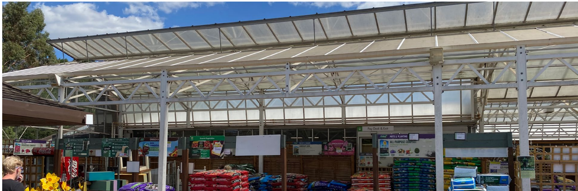
Garden Centre Covered Sales External View
