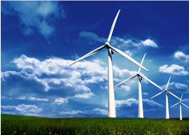
Figure 5. Typical Wind Turbine
