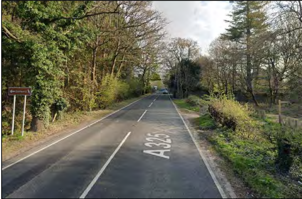
Image 2.14: Footpath 50 Connection with the A325 (Looking North)
