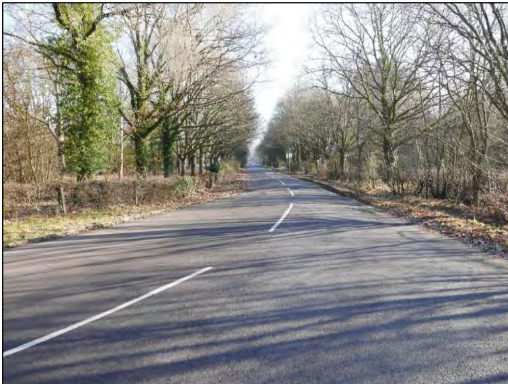
Image 2.7: Gravel Hill Road (Looking East)
