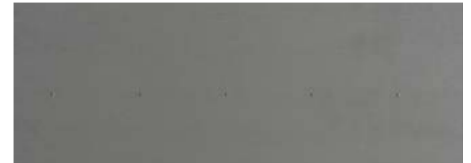
Material: Single Ply Colour: Dark Grey Location: Birdworld Grounds – Roof
