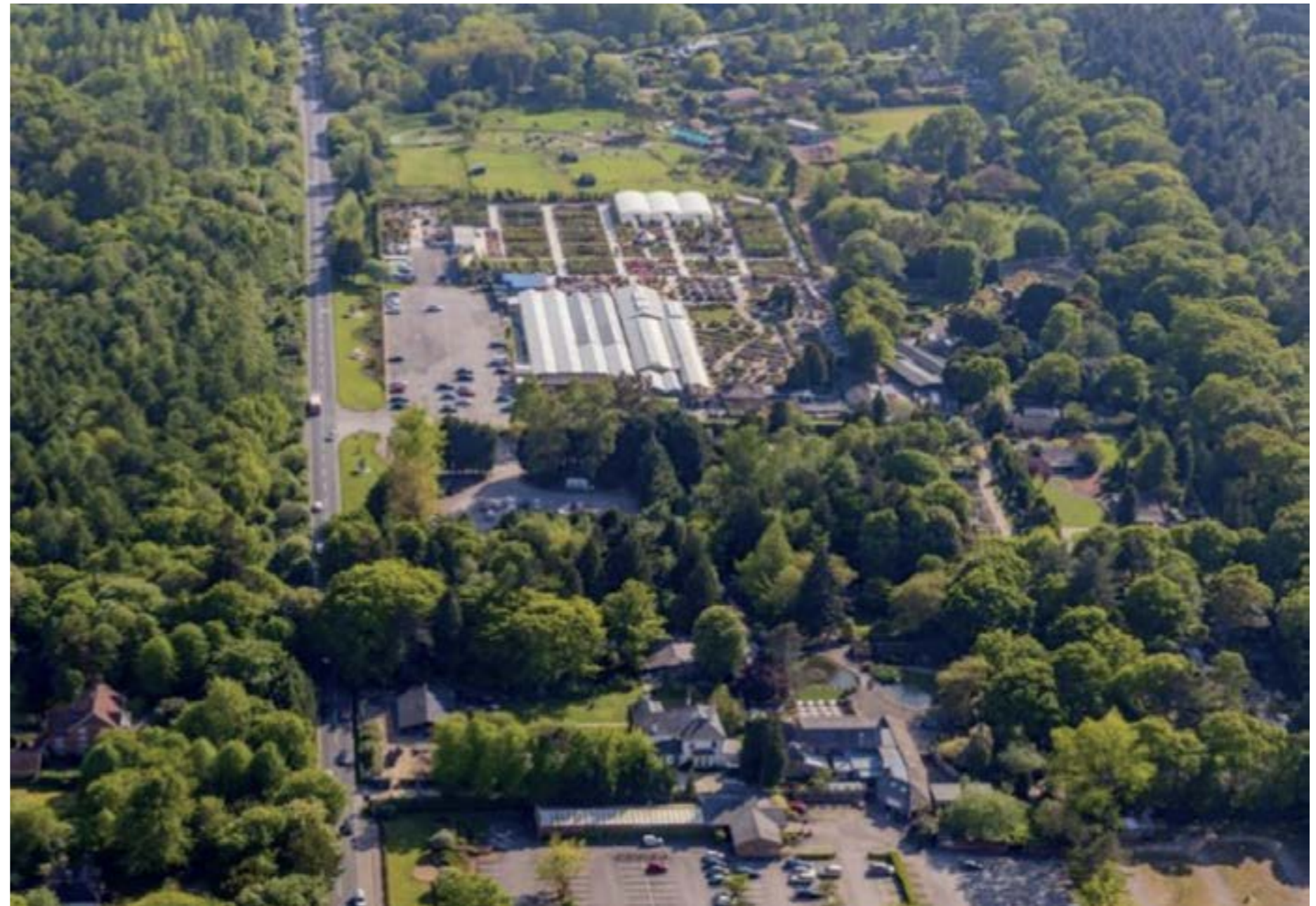
Aerial View of Site
