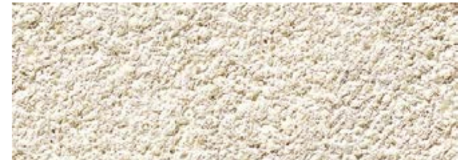
Material: Render Colour: Off-white Location: Birdworld Entrance Building – Walls
