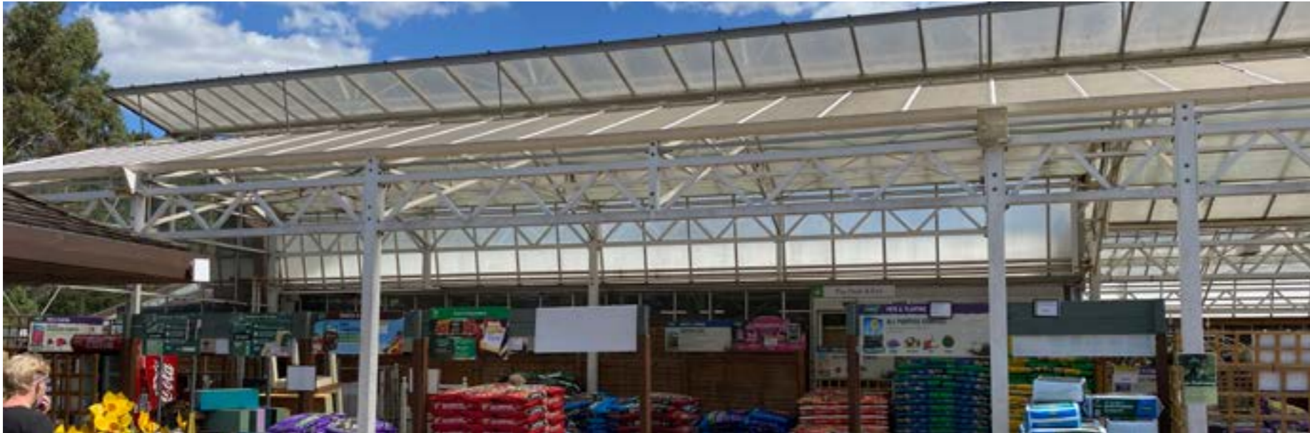
Garden Centre Covered Sales External View
