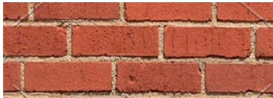
Material: Brick Colour: Red Antique Location: Birdworld Entrance Building – Walls
