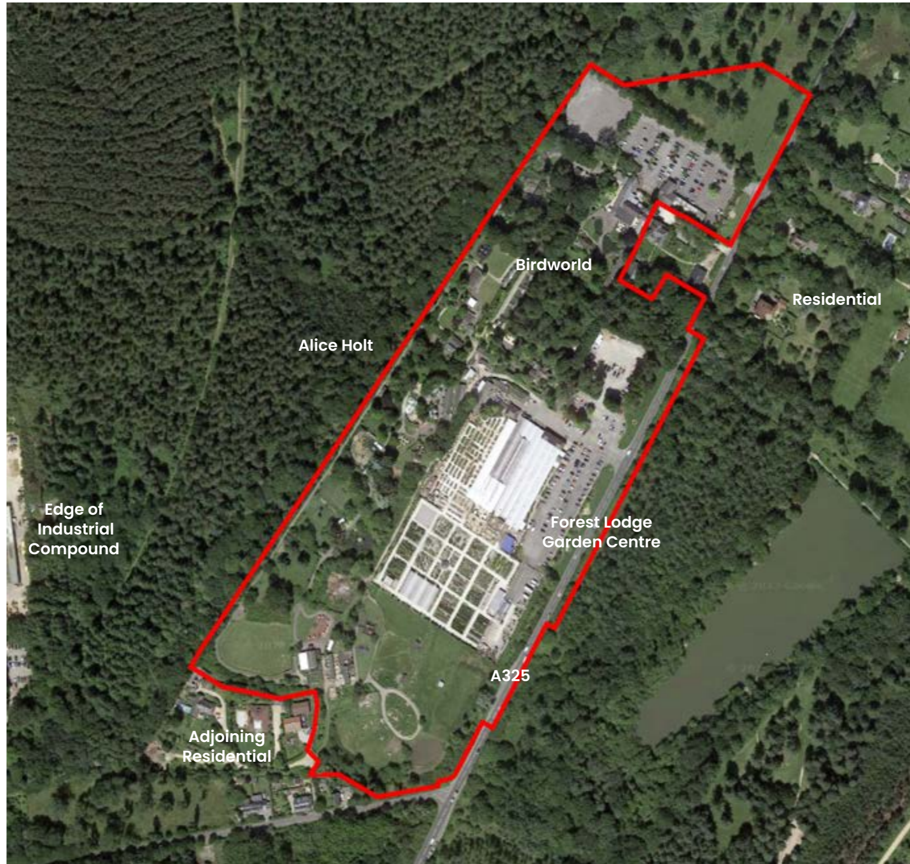
Site Aerial (Ref: Google Earth)
