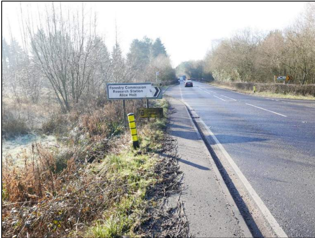
Image 2.4: Southbound Gravel Hill Road Bus Stop (Looking South)
