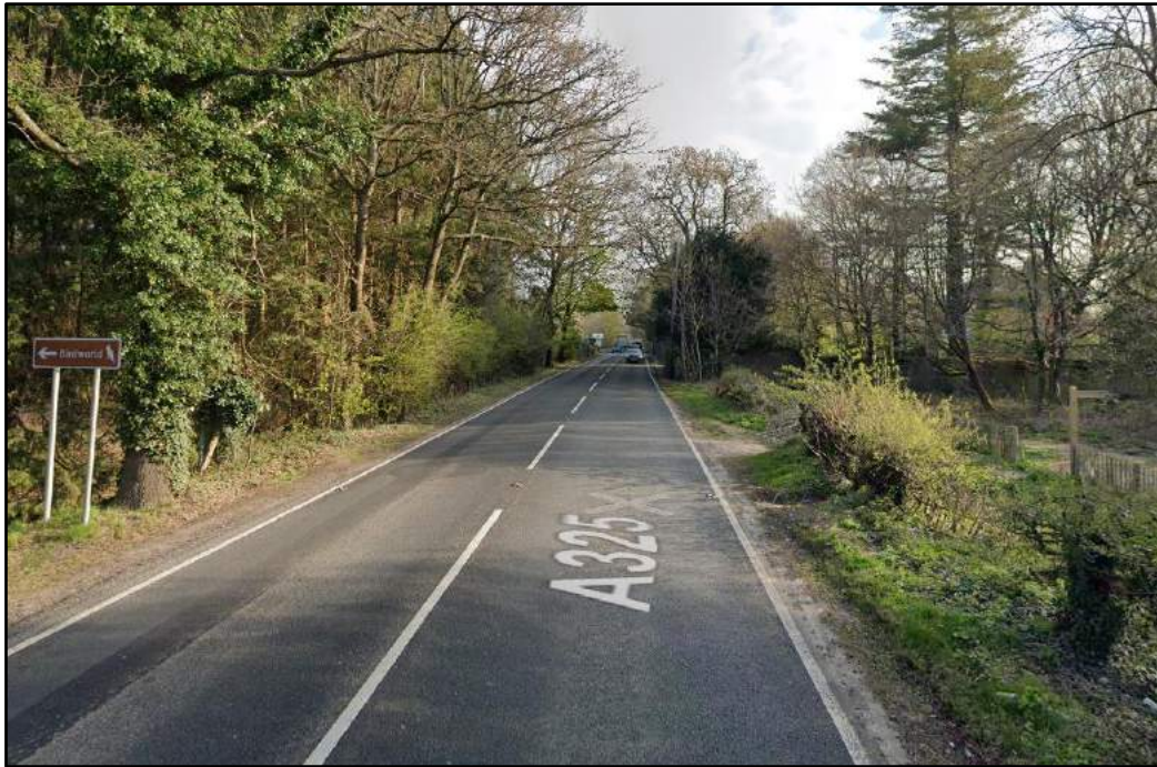
Image 2.14: Footpath 50 Connection with the A325 (Looking North)
