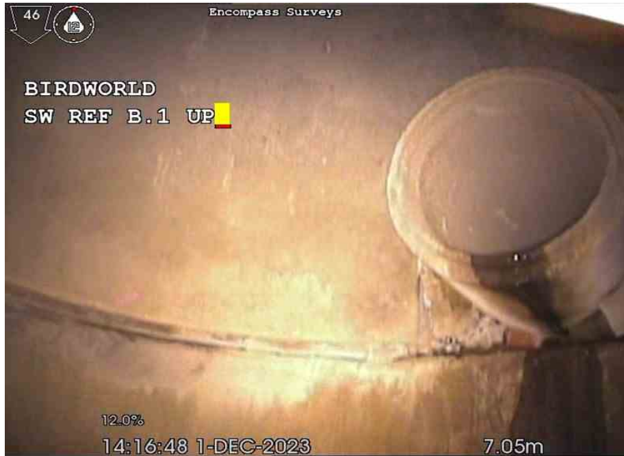
6-1-3A, 00:00:58, 7.05 m Finish node, manhole, reference: MH BURIED
