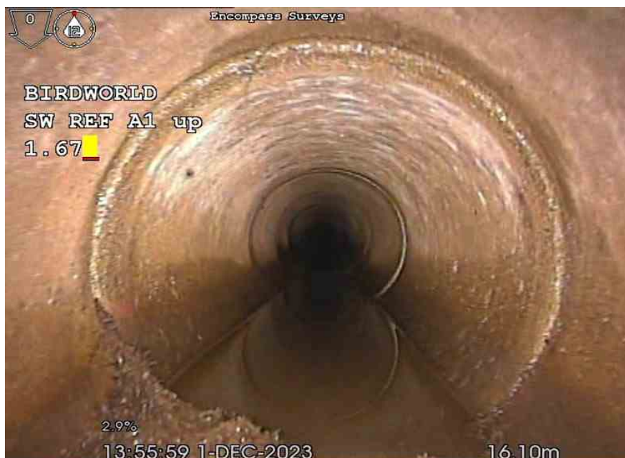
1-1-8A, 00:01:05, 16.10 m Roots, mass at joint, 5% cross-sectional area loss
