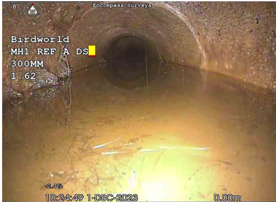
1-2-2A, 00:00:00, 0.00 m Water level, 35% of the vertical dimension
