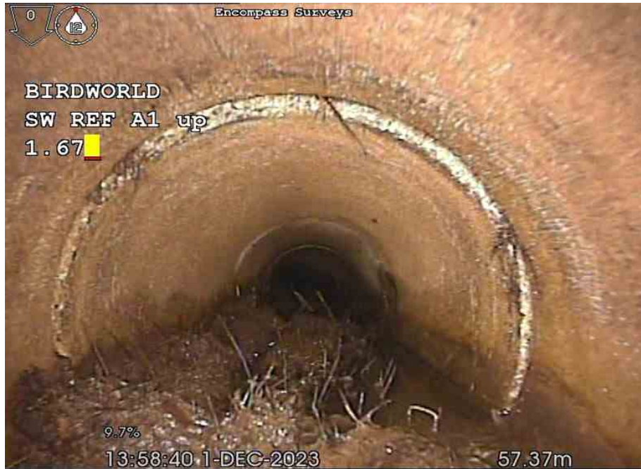
1-1-13A, 00:03:41, 56.28 m Roots, mass, 25% cross-sectional area loss
