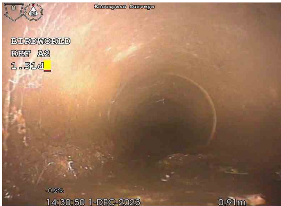
3-1-3A, 00:00:01, 0.00 m Water level, 20% of the vertical dimension
