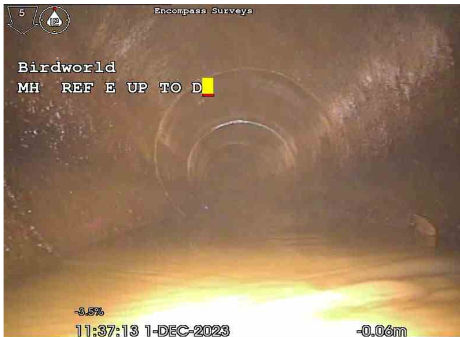
7-1-2A, 00:00:00, 0.00 m Water level, 20% of the vertical dimension
