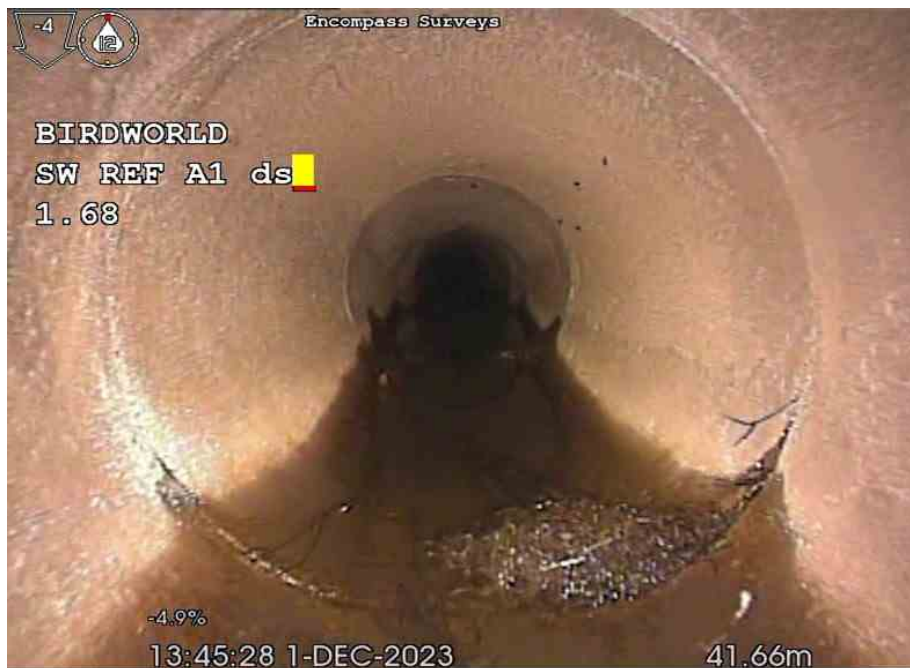
2-1-13A, 00:02:42, 41.66 m Roots, mass at joint, 10% cross-sectional area loss
