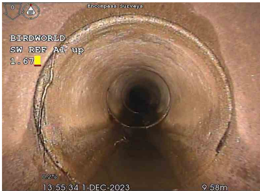
1-1-3A, 00:00:40, 9.58 m Roots, tap at joint
