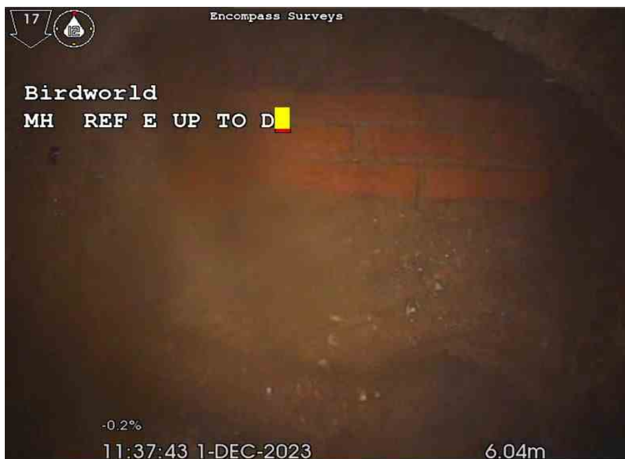
7-1-3A, 00:00:29, 6.04 m Finish node, manhole, reference: MH (D)
