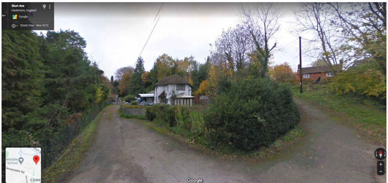
Figure 2 – Private Lane access to the site from the end of Sturt Avenue
