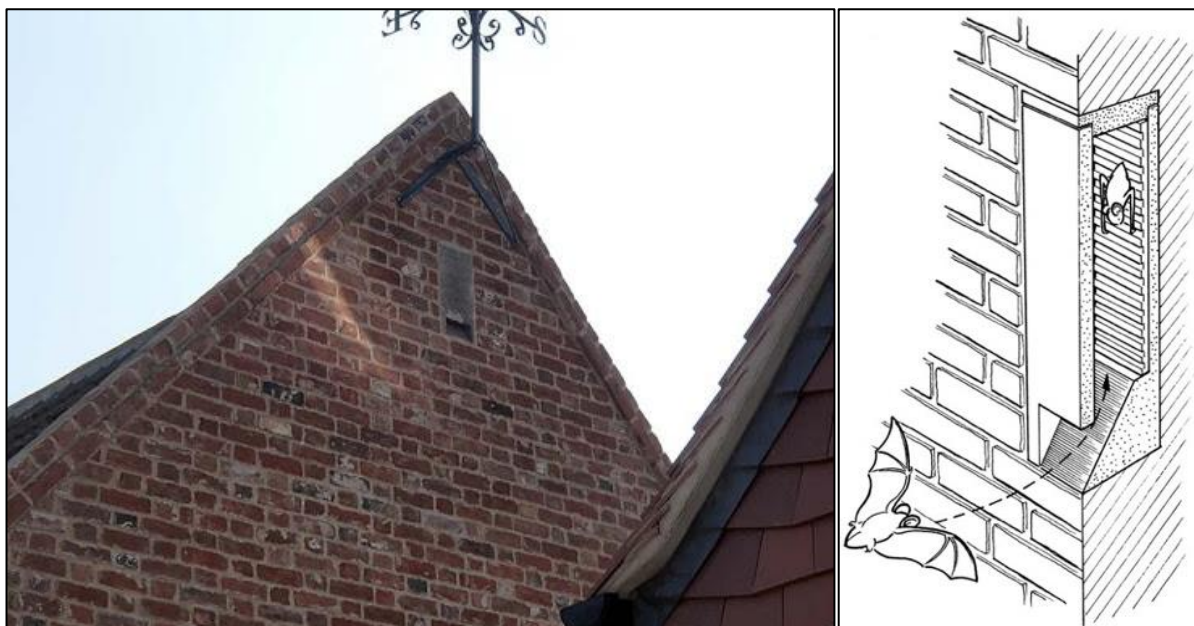
Figure 25. Left – A bat tube integrated into a brick wall. Right – a cross section diagram of a bat tube.
