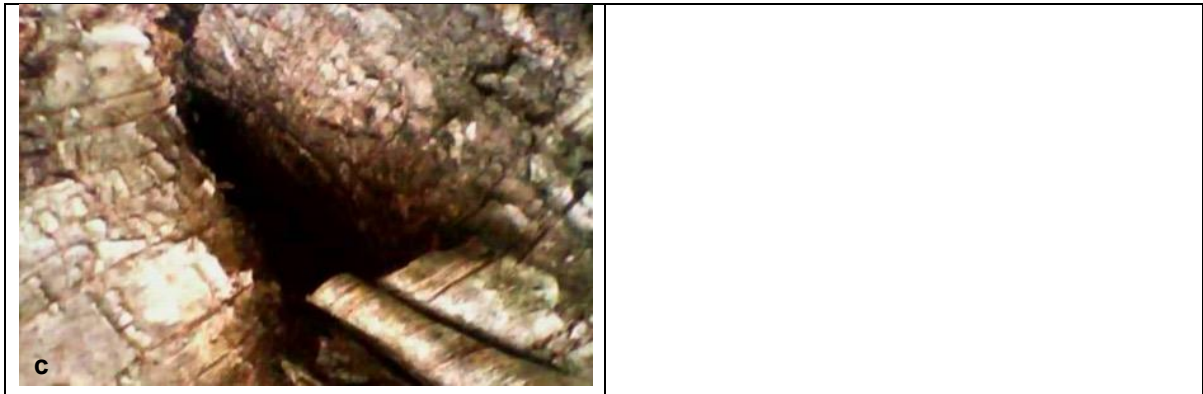
Photographs 9a–c. a – T2. b – a rot hole on the W aspect of the stem viewed from the ground. c – a close-up external photograph of the rot hole.
