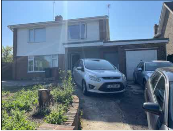
Photograph 1. Western elevation of 1 Carters Way
