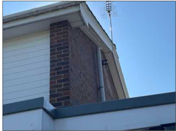
Photograph 4. South-western corner, which is well-sealed
