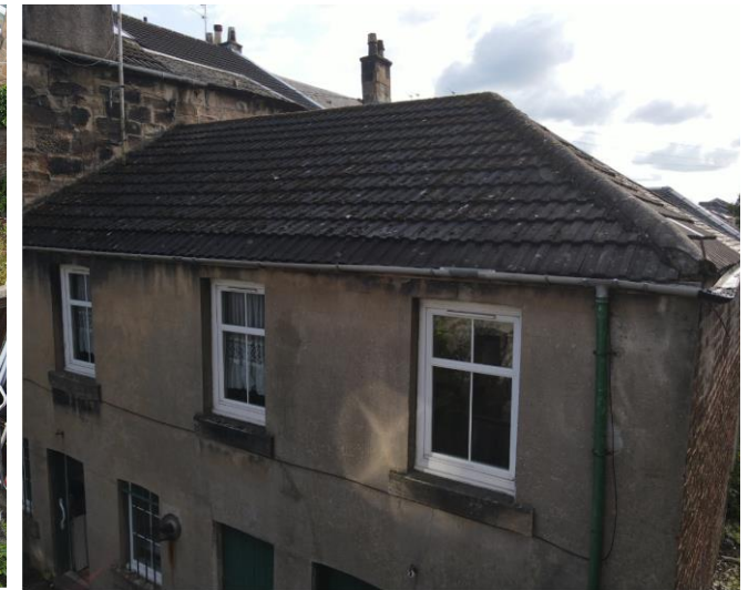
Overview of rear elevations
