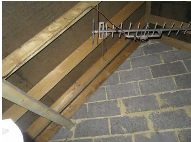
Existing roof looking south
