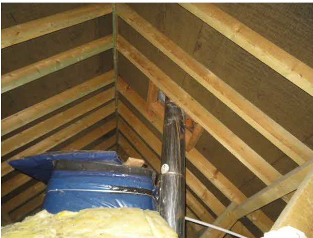
Existing roof looking north towards the flue which will be removed
