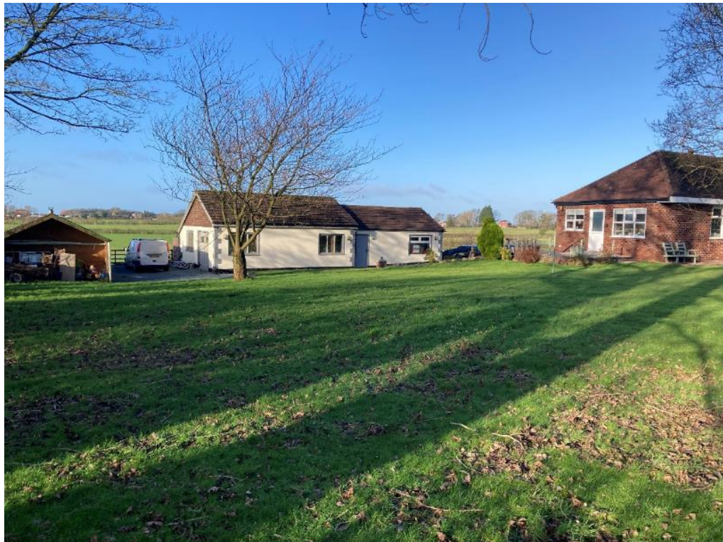
Figure 6: An image of the existing built form on the site
