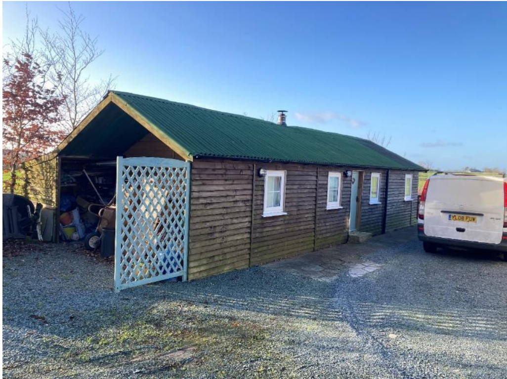
Figure 4: An image of the store room that is to be demolished
