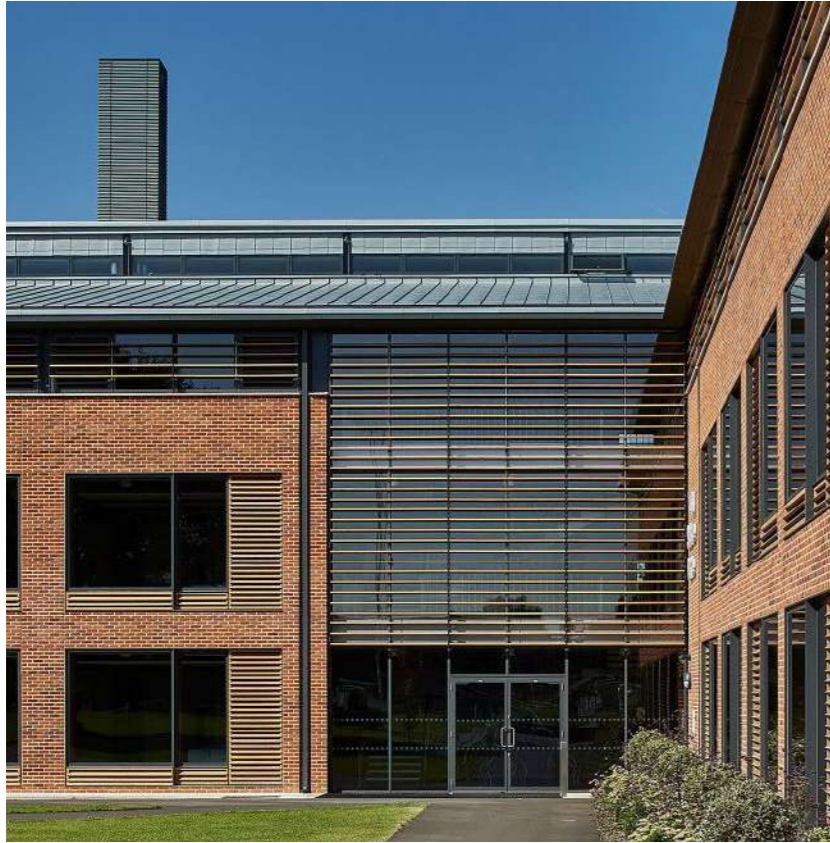
5.08 - Precedent study for timber louvres for attic extension - Abingdon School by Ridge and Partners LLP
