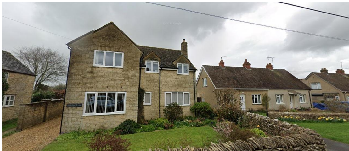
Properties immediately north of the application site (Google maps)
