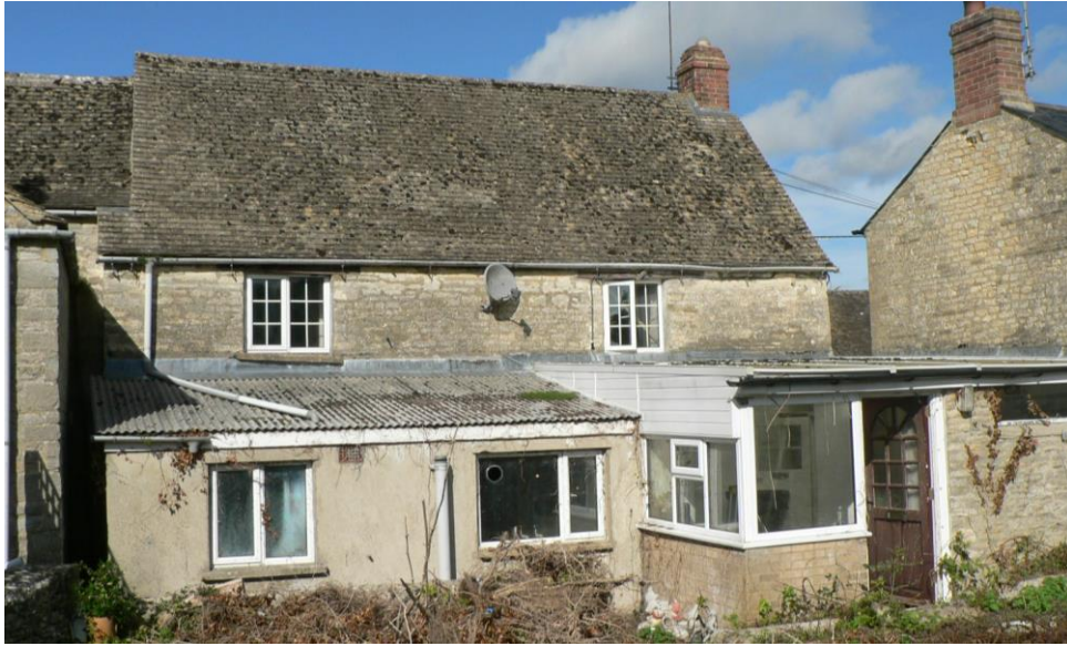
Existing rear elevation of 28 Lower End
