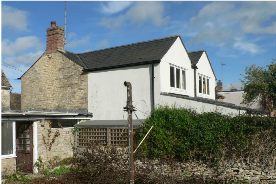
Existing rear elevation of 30 Lower End
