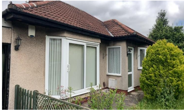
Photo 2 Building on site
