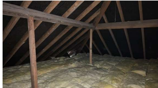
Photo 10 B1 (loft void)
