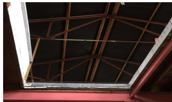
Photo 12 B2 (roof interior)
