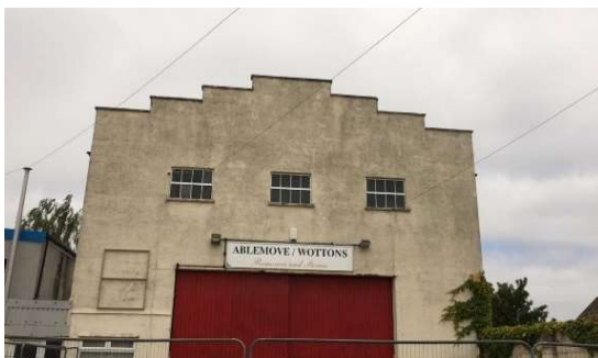
Photo 11 B2 (southern elevation)
