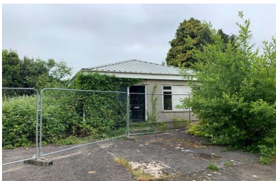
Photo 13 B3 (southern elevation)
