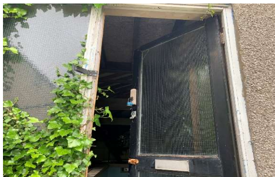
Photo 14 B3 (roof interior)
