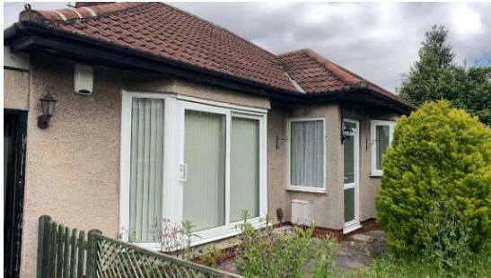
Photo 9 B1 (southern elevation)
