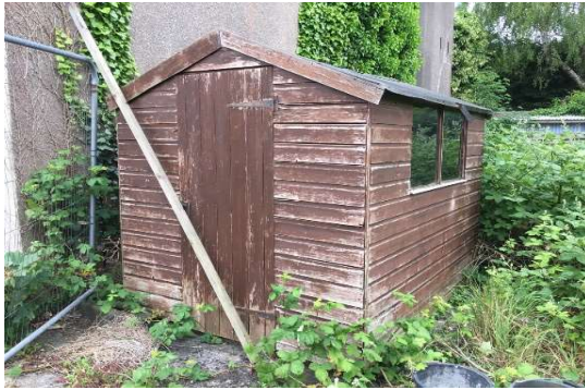
Photo 13 B4 (southern elevation)
