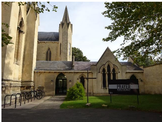
Photo 05 General view of Hall elevation from Malvern Road (September 2023)
