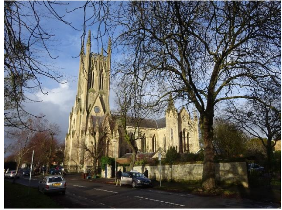
Photo 02 General view of southeast elevation from Malvern Road (December 2023)
