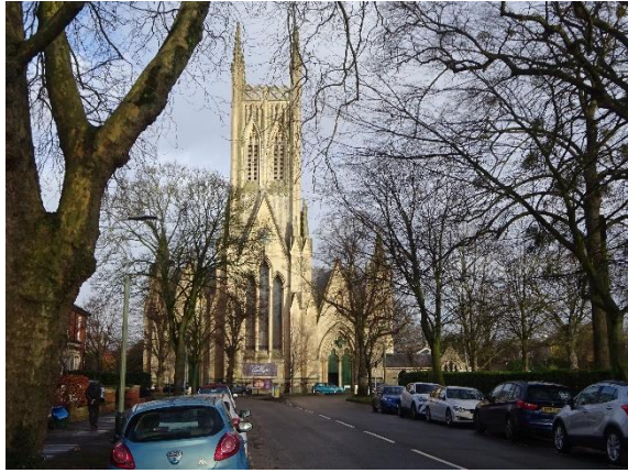
Photo 01 General view of southwest elevation from Christchurch Road (December 2023)
