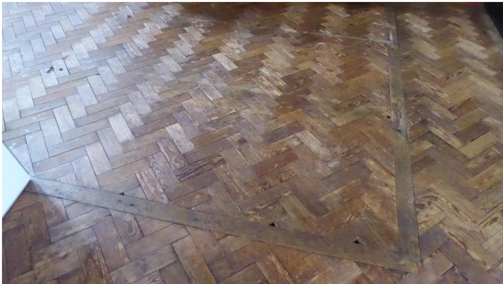
Figure 51 Parquet floors characteristic of much of the interior – here also showing evidence of the position of former pews that have been removed
