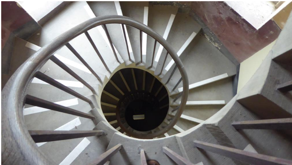
Figure 30 South Transept gallery stairs
