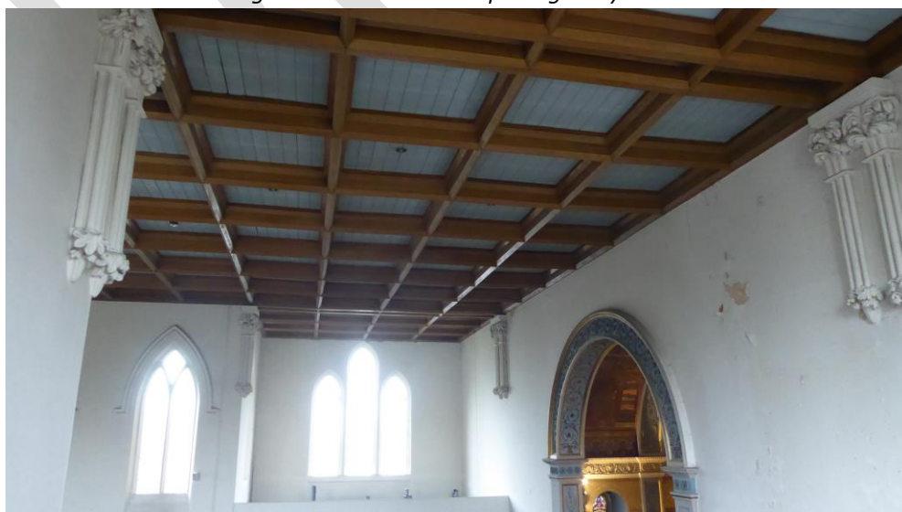
Figure 29 View across transepts showing clustered shafts with Gothic style foliage carving
