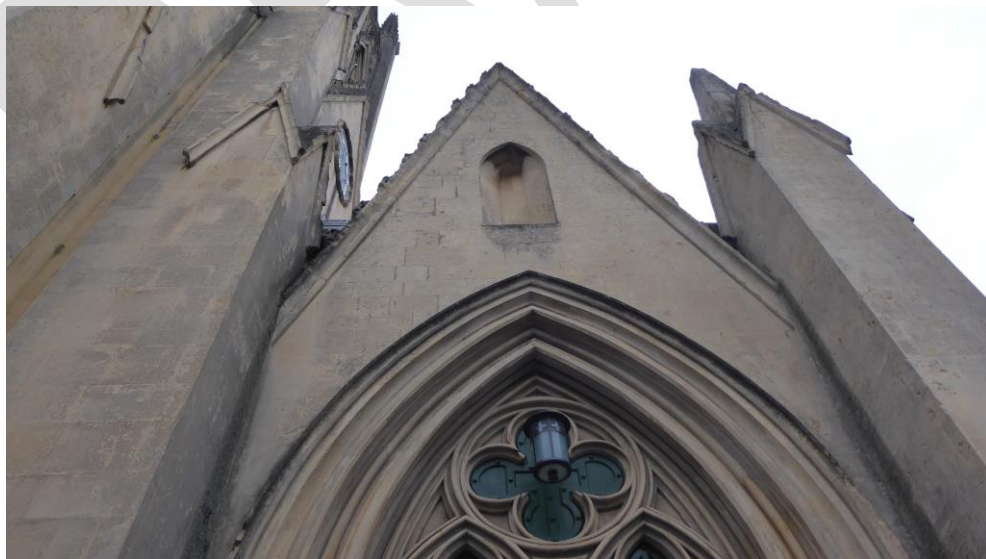
Figures 61 and 62 Evidence of stonework erosion
