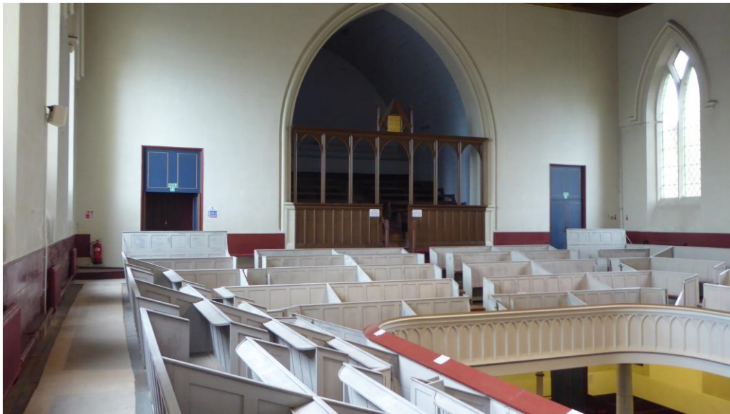
Figure 19 View west from the south gallery
