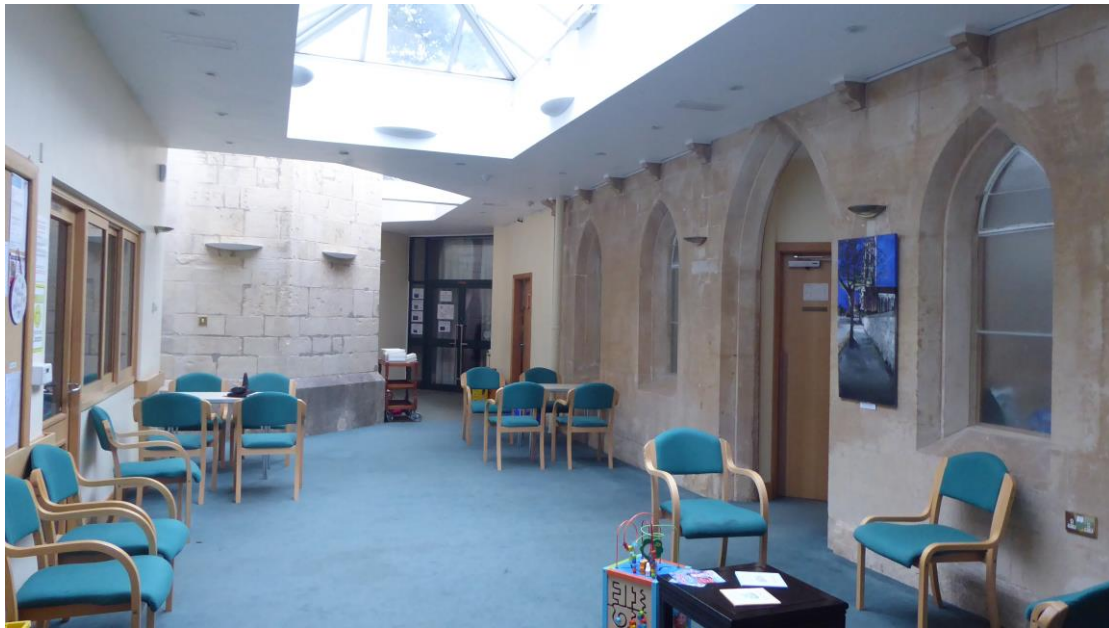
Figure 58 View east through the covered space created between church and former school
