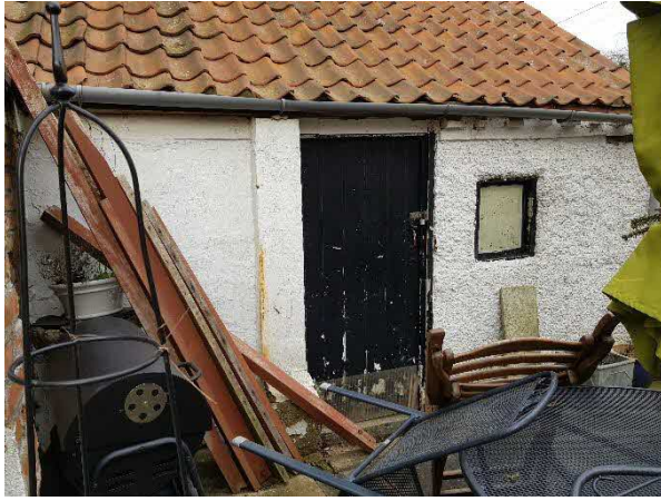
Figure 28 Southern elevation of the barn. A blocked arched opening formerly containing flight holes for a dovecote is located in the upper gable end of the south elevation (R) and there is a single storey monopitch structure on the south side of the gabled elevation (L).
