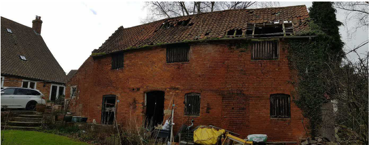
Figure 27 Panoramic view of the east elevation of the barn.
