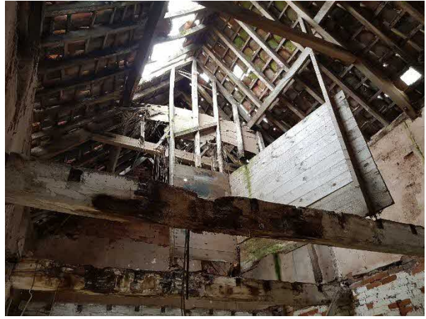
Figure 34 Looking south within the main southern space showing upper floor removed.
