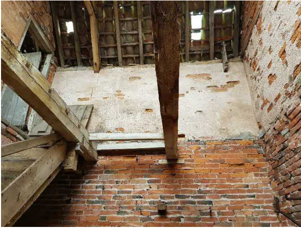
Figure 31 Looking west within the northern space.
