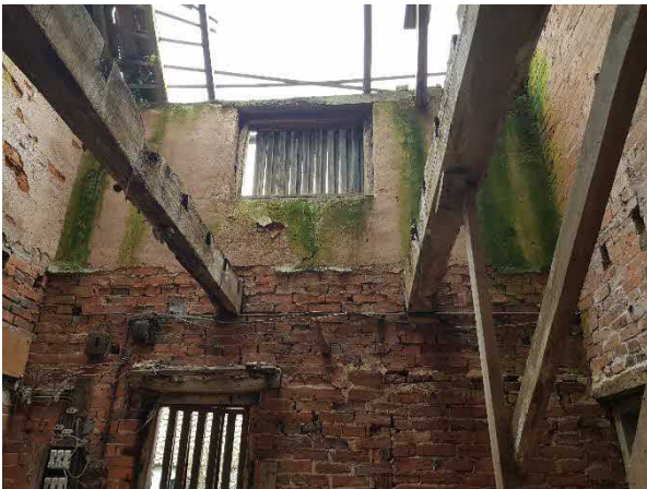
Figure 33 Looking east within the northern space.
