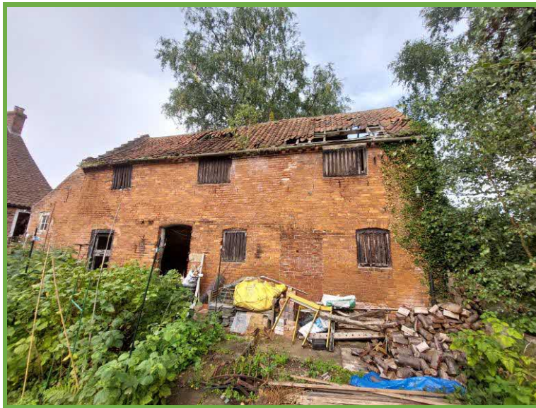
Photo 1: View of the detached barn (eastern aspect)
