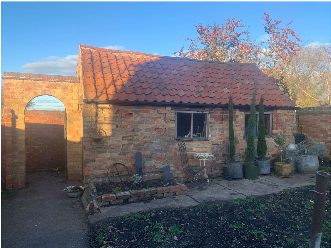
Photo – existing piggery out building
