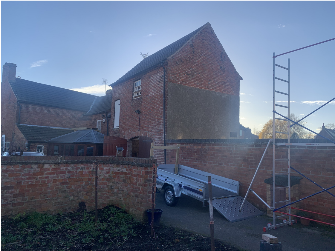
Photo – existing Dovecot to the rear of the dwelling
