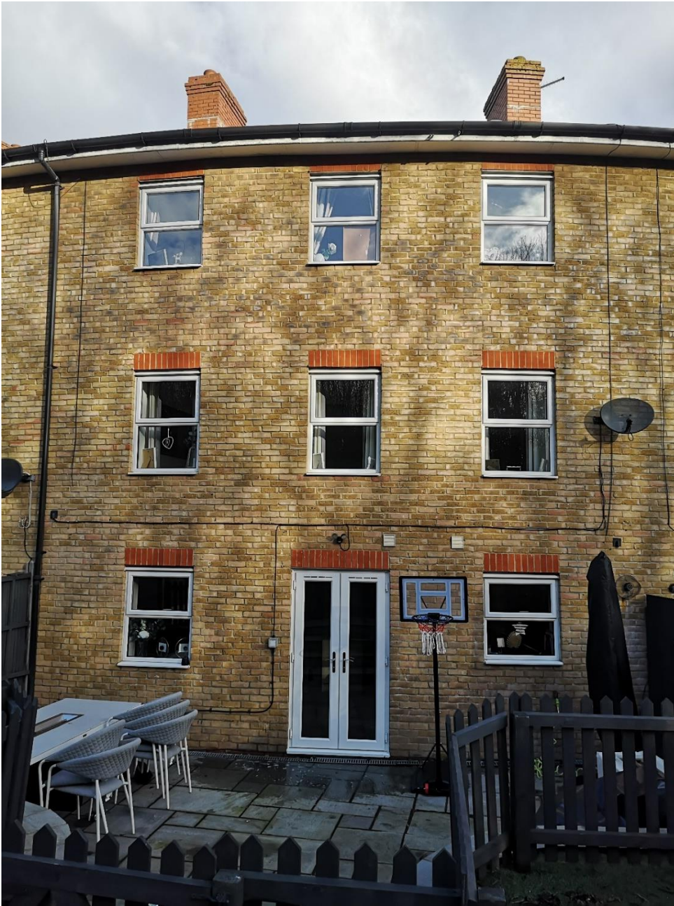
1. View of existing rear elevation
