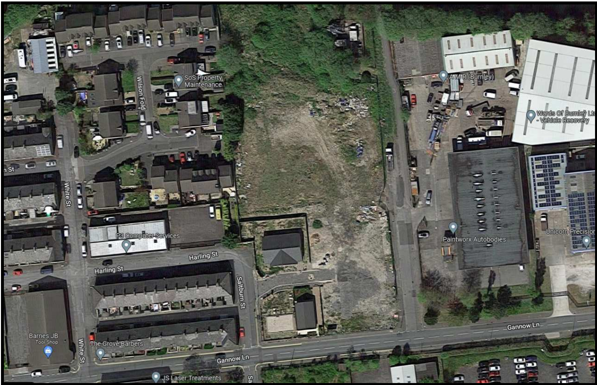
Site with 2 units from previous approval constructed and now demolished
