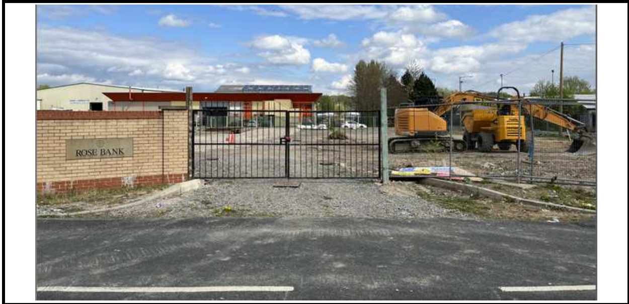
Existing site access
