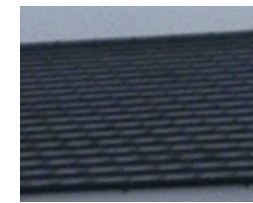
1. Natural slate roof
