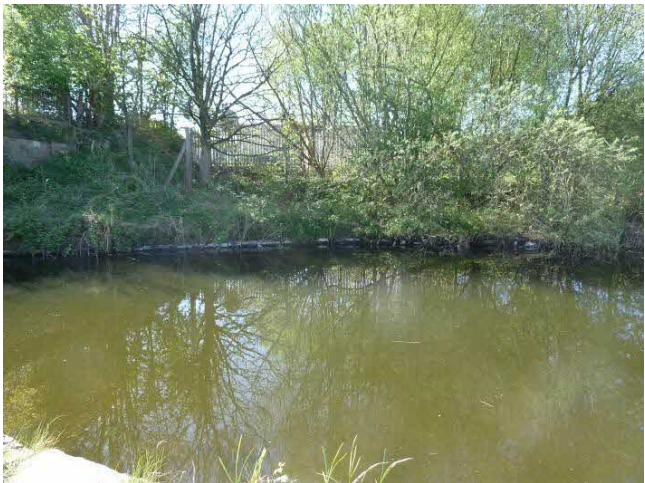
Photograph 16: The canal margin adjacent to the site – hard stone revetments exposed.
