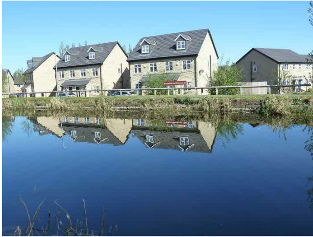
Photograph 17: The towpath side of the canal with exposed stone revetments and scattered marginal stands.
