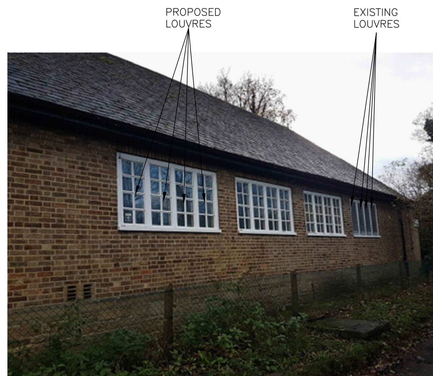
PHOTO OF WEST ELEVATION
