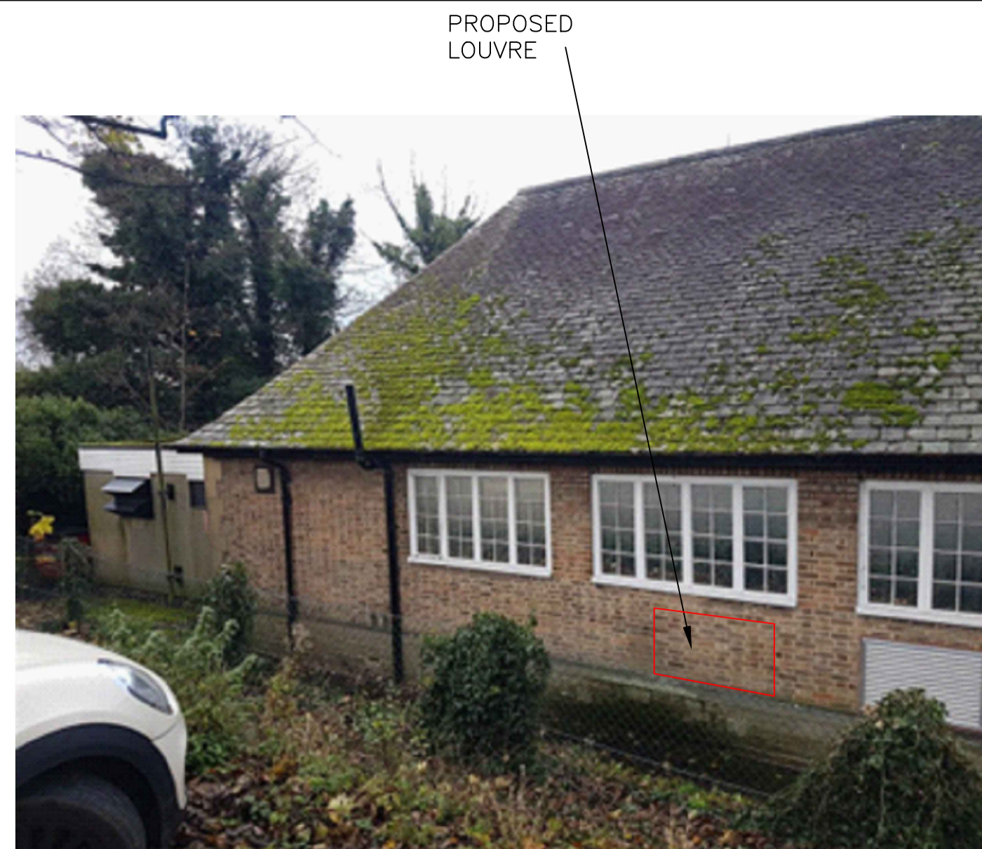
PHOTO OF EAST ELEVATION
