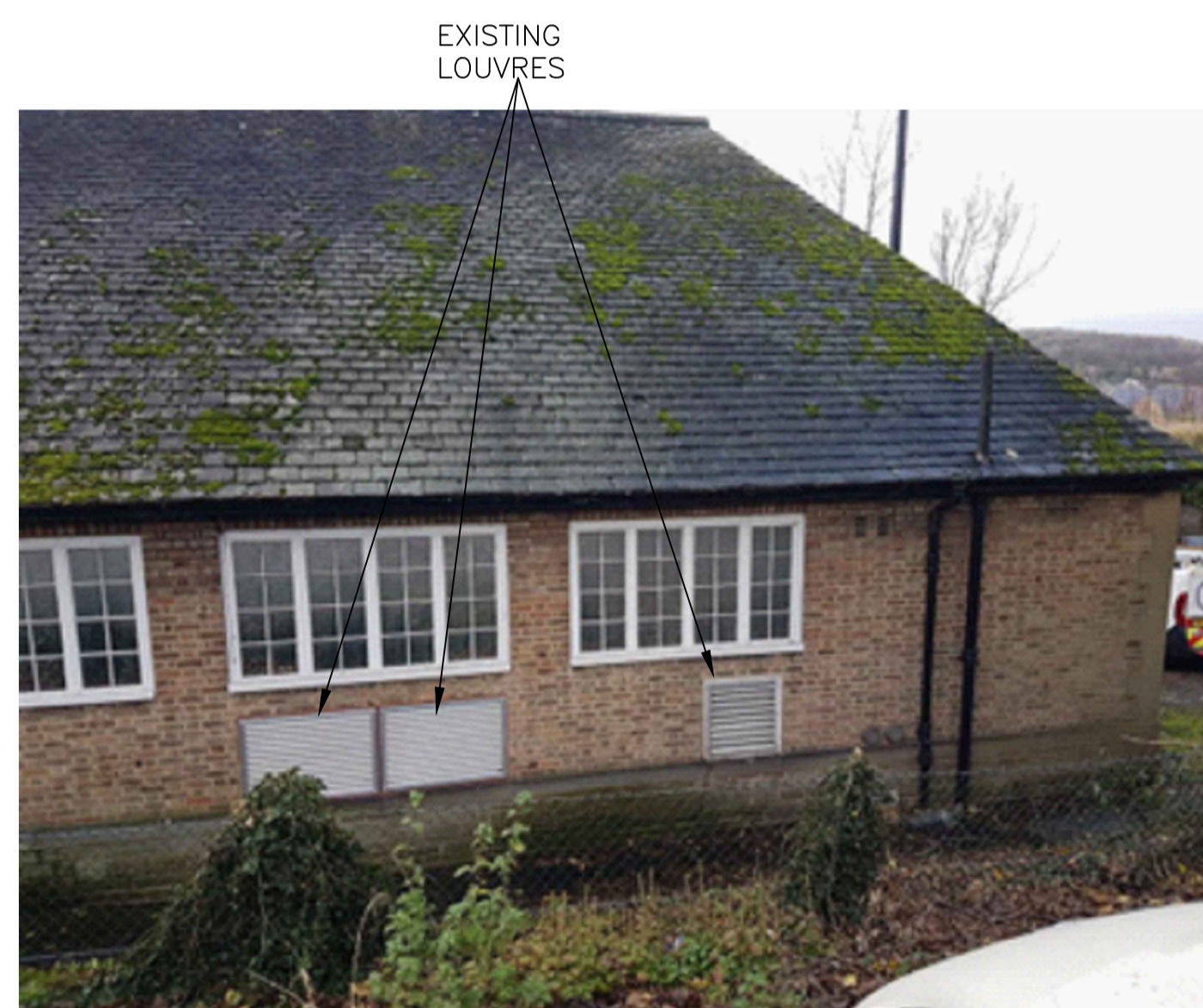
PHOTO OF EAST ELEVATION
