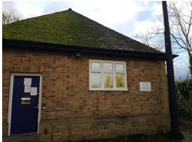
SOUTH ELEVATION – OPPOSITE STATION ROAD
