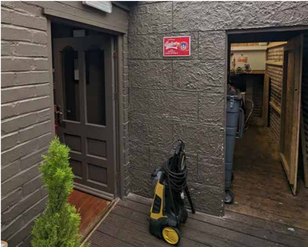
Above: photo taken within entrance lobby area, facing east illustrating existing late-C20th timber framed entrance door and bin store stud wall featuring faux stone plaster to wall.
