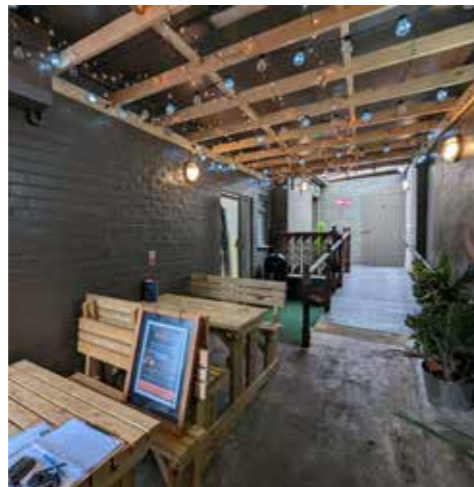
Above: photo taken within ground floor lobby area, facing west.
