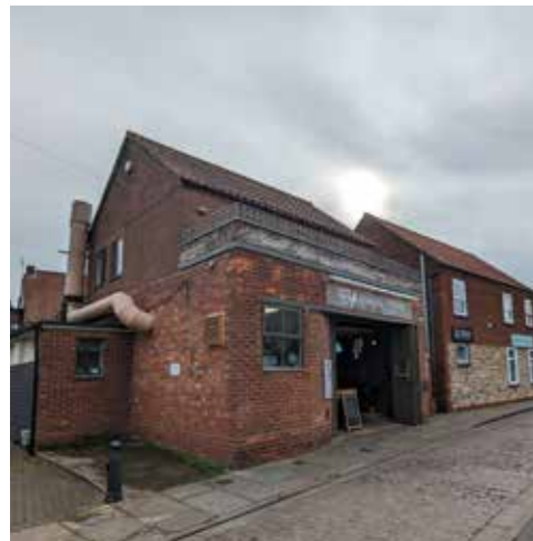
Above: photo taken of external front elevation, facing south-east.
