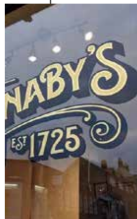
Manifestation signage to new glass panel entrance door.
