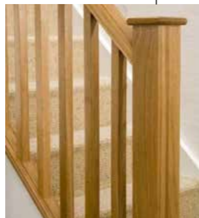
Oak timber square spindles and newel posts to existing ramp.
