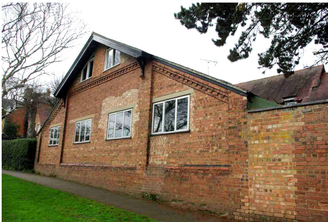
Figure 19: Northern end of Meadhurst extension seen from Ayston Road
