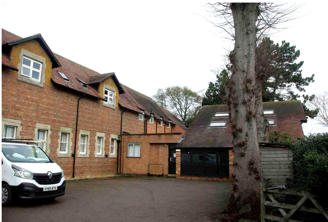
Figure 18: East facing Meadhurst extensions
