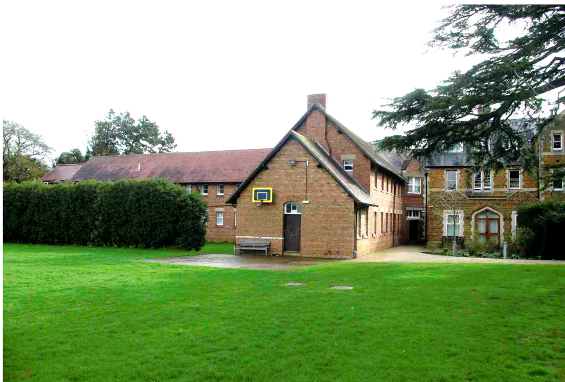
Figure 26: Rear view of Meadhurst
