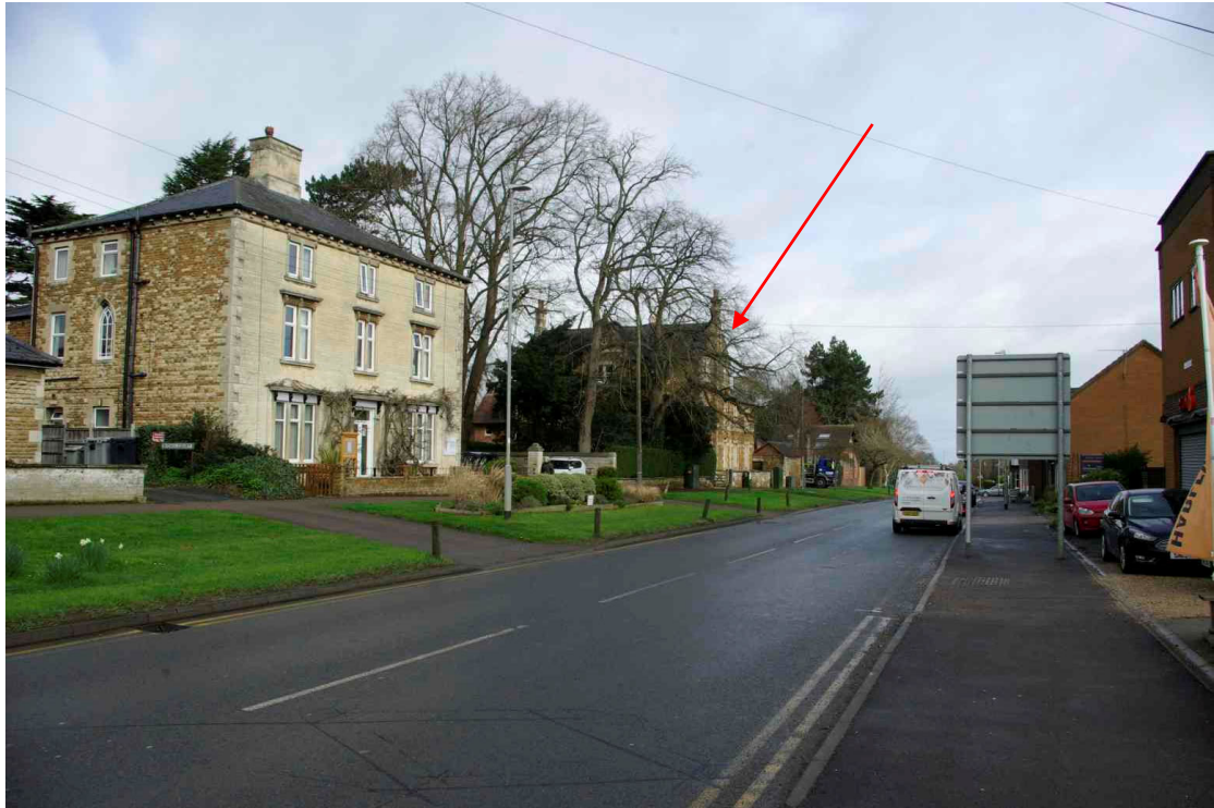
Figure 14: Meadhurst site seen from Ayston Road Looking north-east. Stone-built part of Meadhurst arrowed
