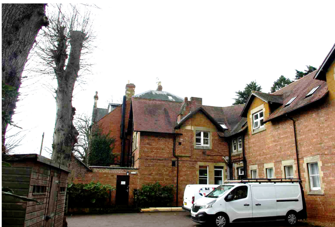
Figure 17: East facing Meadhurst extensions Looking south. Ayston Road on the right
