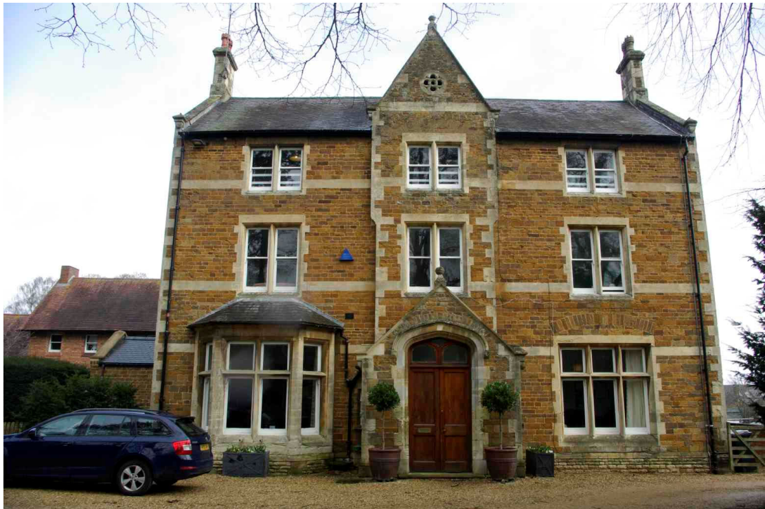
Figure 21: South facing elevation of Meadhurst Looking north at the original part of the building. Ayston road to the right
