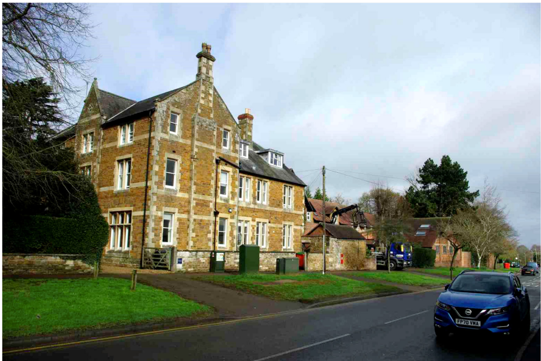
Figure 15: Meadhurst seen from Ayston Road Looking north-west. The original stone-built component is on the left, later brick-built extension runs to the north on the right of the picture
