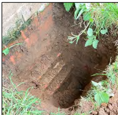
Photo 2 - A photograph showing the thickness of foundations within FP02.
