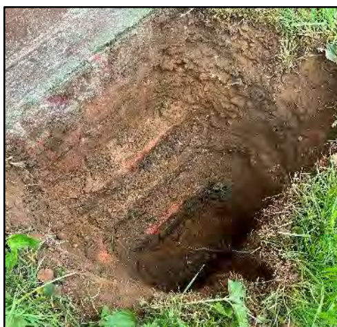
Photo 1 - A photograph showing the thickness of foundations within FP01.
