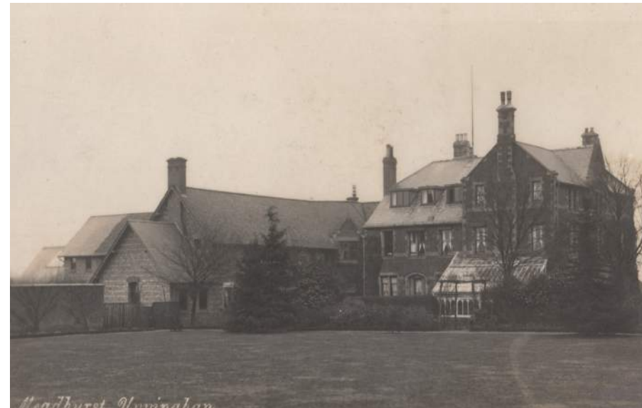
1910 Roofspace within rear section of original house converted, dormers added. Single storey extension to dormitory wing,
