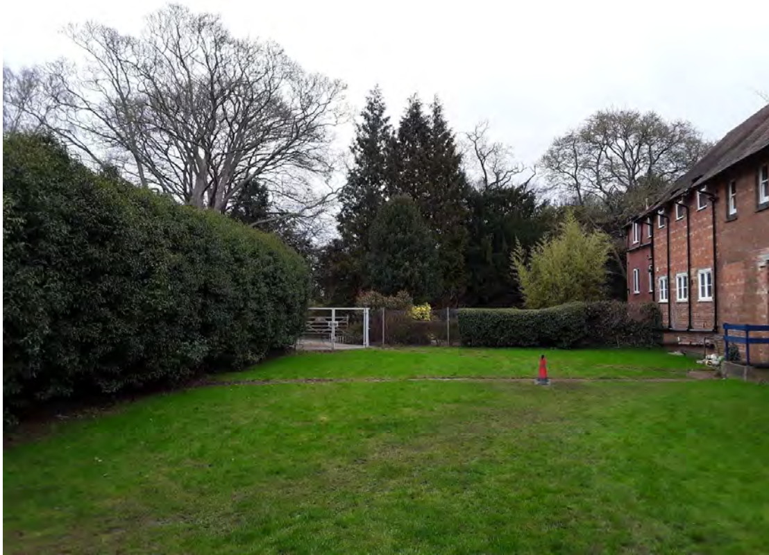
Figure 3 – Looking northwards with H3 to the left of the photo and the existing building to the right.
