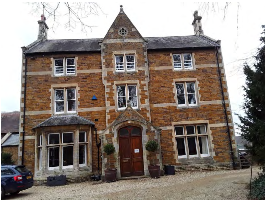
Figure 1 – Looking northwards at the existing building.
