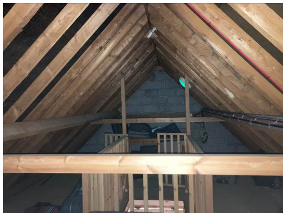
Interior loft of section B
