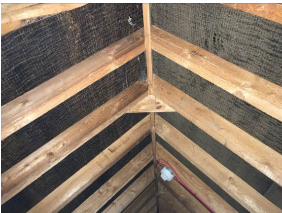
Interior loft of section B
