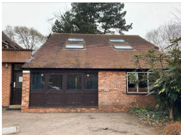
South face of section C
