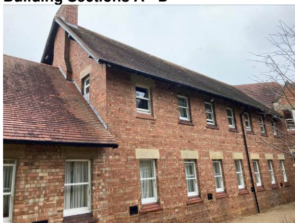
South face of section A
