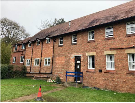
West face of section B
