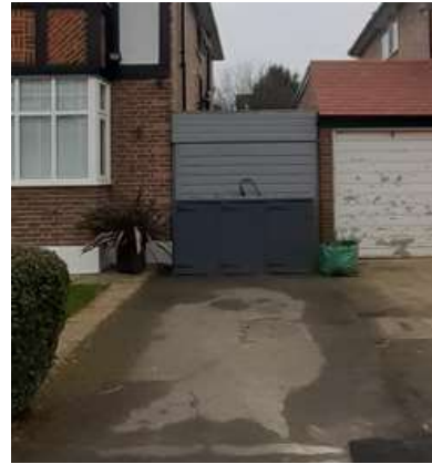
Existing parking drive-in and neighbours side extension.
