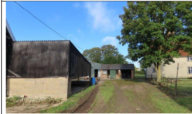
Area north of traditional barn (building 3). Building 6 is visible centre and building 7 is to right of image.
