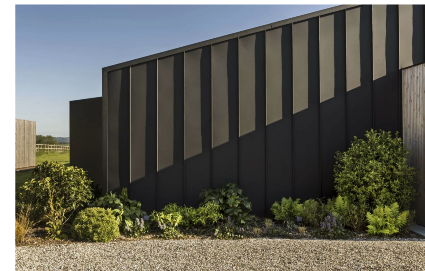
CRINAN BARN BY HOLLAND GREEN CLADDING EXAMPLES
