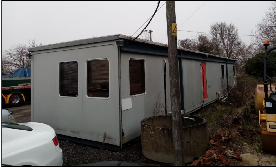
Figure 2.4 Rear Elevation of office
