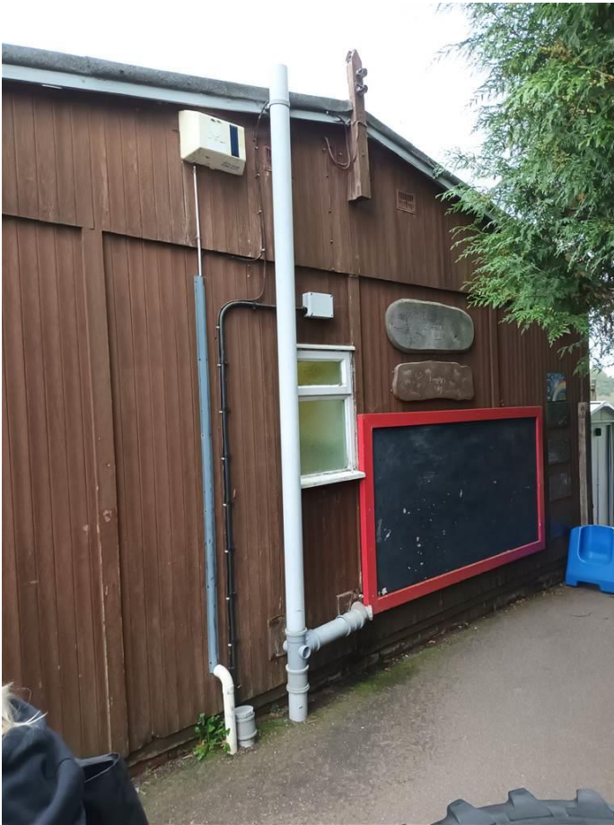
Fig 1.2. South elevation existing timber frame classroom.
