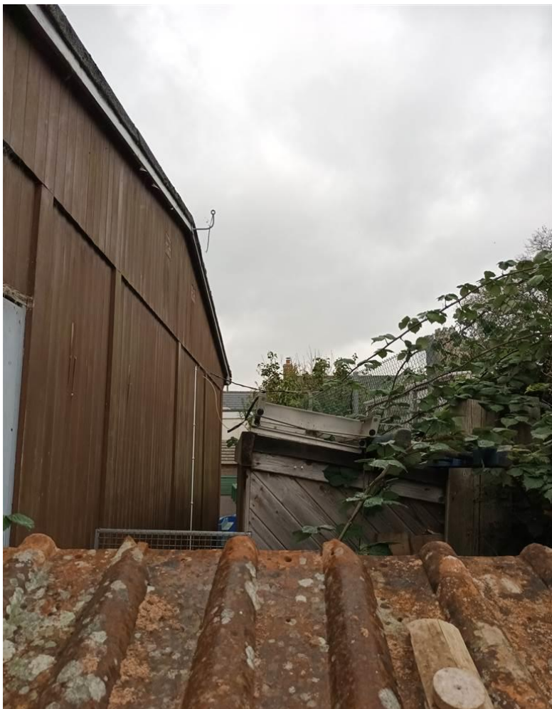
Fig 1.3. East elevation existing timber frame classroom.
