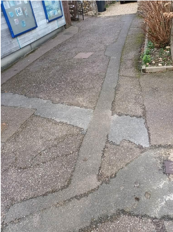
Fig 1.6. Road access to neighbouring property between main school building and classroom.
