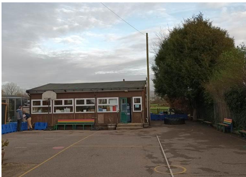
Fig 1.1. West elevation existing timber frame classroom as viewed from the playground.
