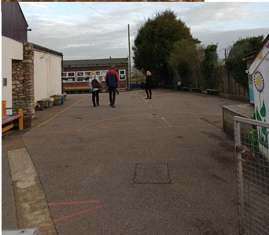
Fig 1.4. North elevation existing timber frame classroom.
