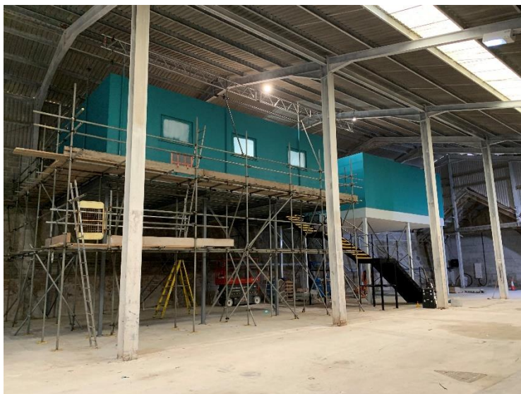
Linhay Building – Mezzanine level, laboratory and visitor centre
