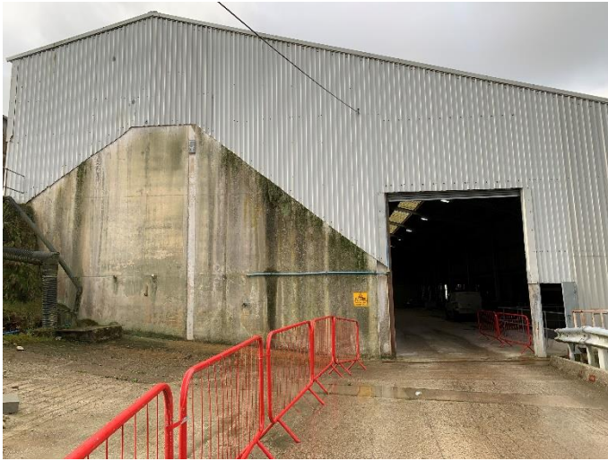
Linhay Building – East elevation, main entrance
