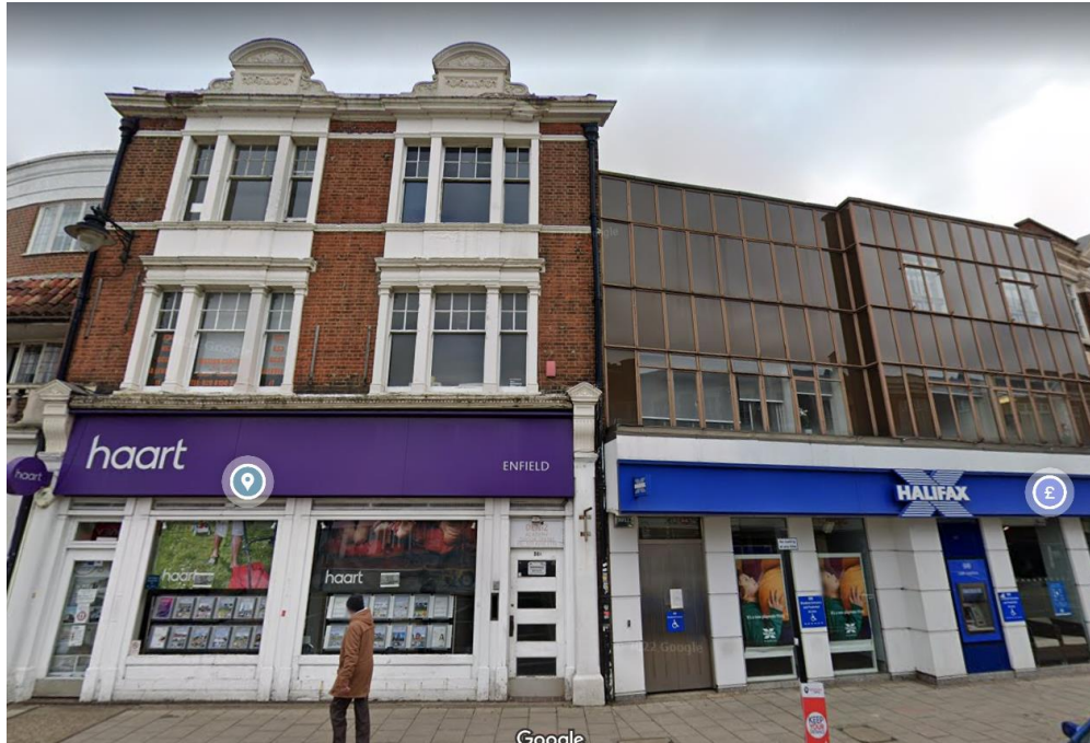
(fig 7- The surrounding built form (London Road) which defines the era the property was built)
